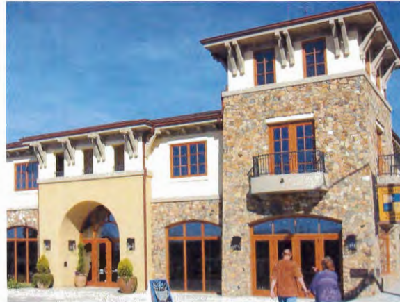
This building has a formalized tower element at the street corner. The tower is a full story taller than the remainder of the building and its facade slightly extends beyond the adjacent building facades to further accentuate the corner.
