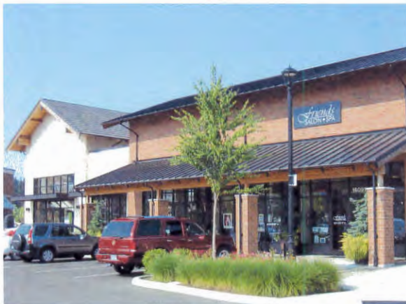
This storefront building in Happy Valley faces a sidewalk in a commercial development. The gallery provides shelter and adds visual interest.
