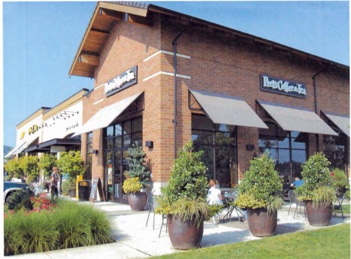
The corner building of this multi-tenant development is clad in brick and provides a contrast to the stuccoed facades.
