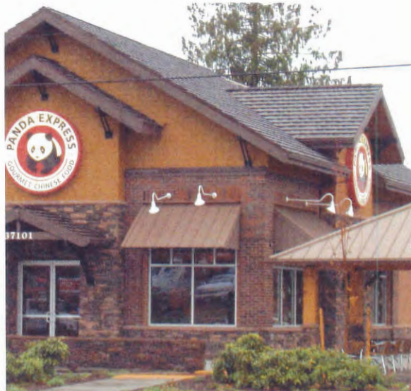
The base of this building is clad in multi-colored brick, which provides a nice contrast to the wood cladding above.
