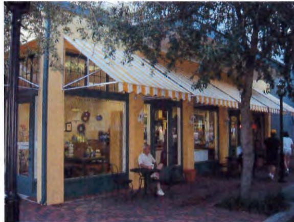
This traditional storefront building has all the elements of pedestrian-friendly design: large transparent windows, awnings, doors that open directly on the sidewalk, sufficient room for outdoor seating and merchandise display, and street trees that do not block views.
