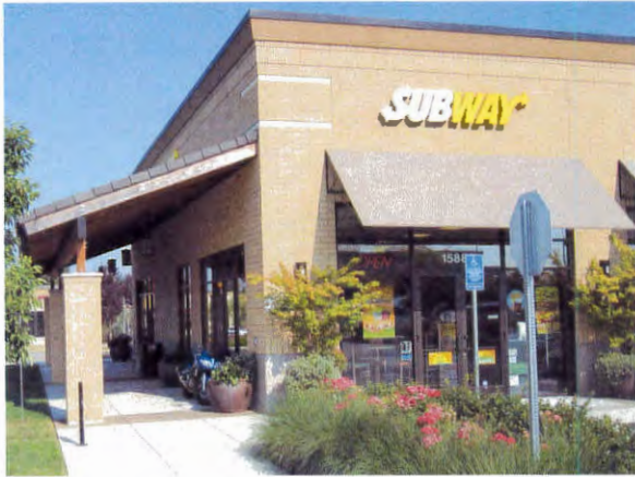
A brick clad wing of a building in Happy Valley utilizing yellow brick as primary material.
