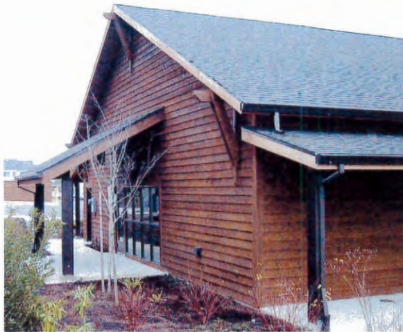
The Hikade building incorporates a variety of materials that exemplify the Happy Valley Style, including stone (primary material), wood, glass and steel. The building's side wing is clad in wooden lap siding, evocative of a barn structure.
