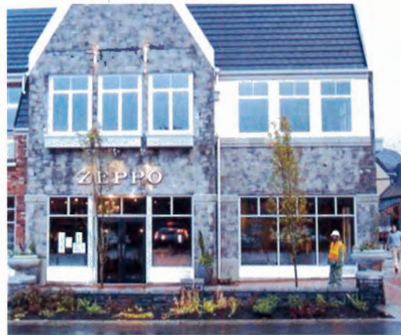
Lakeview Village (Lake Oswego, Oregon) uses rusticated stone as the primary building material for this portion of the office retail development.
