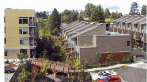
As part of the Headwaters development in Portland, Oregon the buried Tryon Creek was daylighted and restored to a naturalistic condition.
