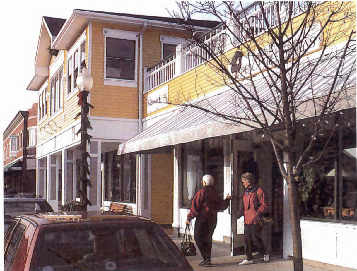
This commercial storefront building in Mashpee, Massachusetts is located at the sidewalk and has entrances at the front, thus activating the street facade and creating a lively an interesting street experience. The awnings and arcade provide shelter from rain and sun a add to the pedestrian experience.
