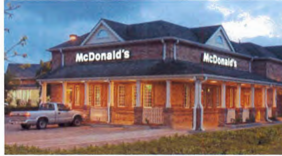
This fast-food restaurant has a flat roof with an applied pitch, intended to appear like a pitched roof. The roof line is further varied by gable ends that break up the applied pitch, and by a gallery structure attached to the building facades.
