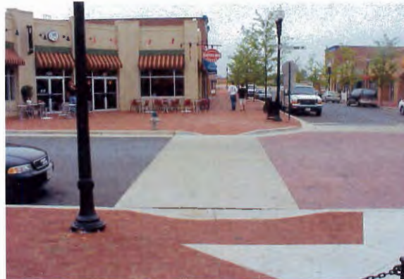
Textured and colored sidewalks and crosswalks can provide visual cues to drivers and help improve pedestrian safety. They can also contribute to an aesthetically cohesive development.
