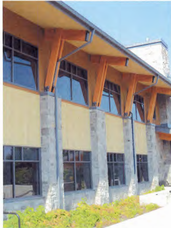
Happy Valley’s new City Hall uses a combination of stone cladding, wood siding and structural elements, and generous amounts of glass to create an interesting facade pattern.
