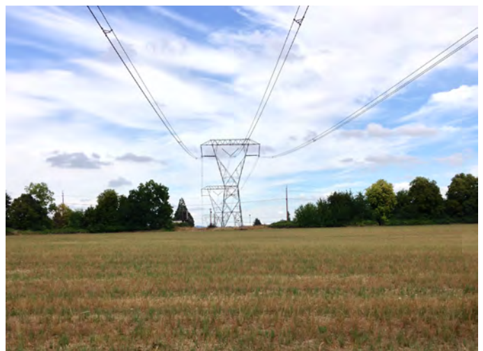
Bonneville Power Administration lines through South Hillsboro.
