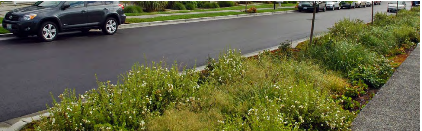
Bioswales in a residential development treat stormwater runoff from the street and sidewalk
