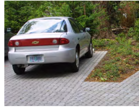
Sustainable design - permeable parking surfaces
