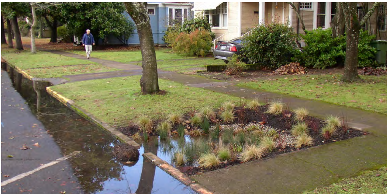
Figure 25 Bioswale on Court Street NE
