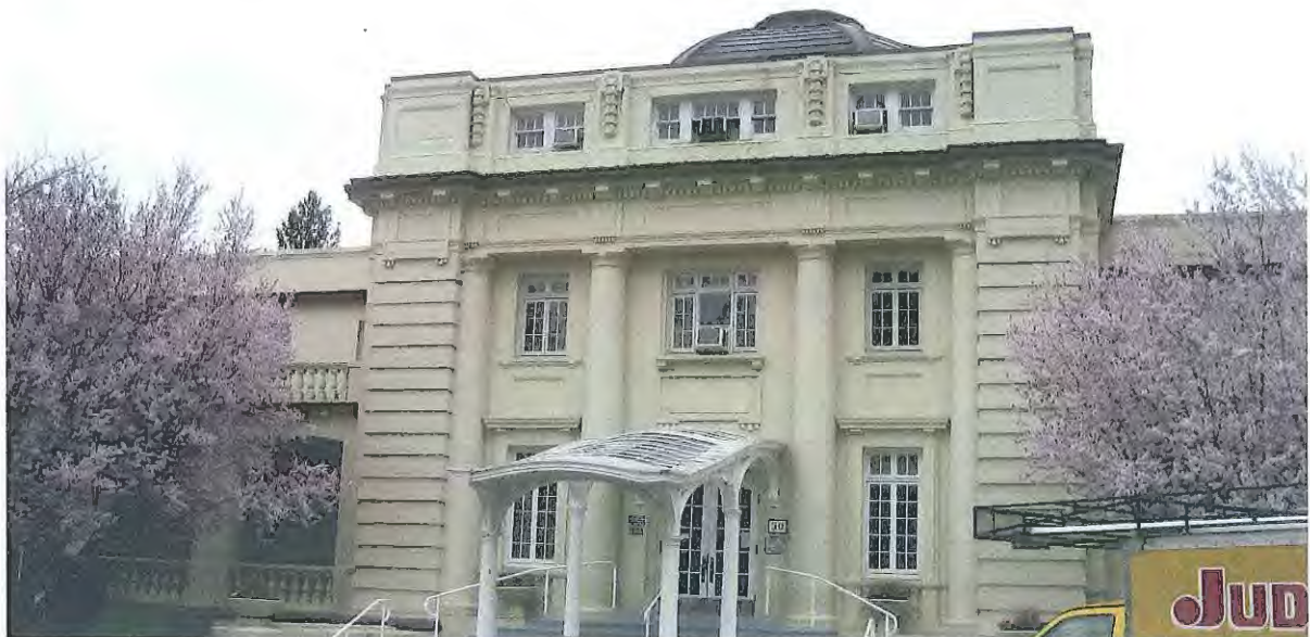
Figure 38 Historic Dome Building
