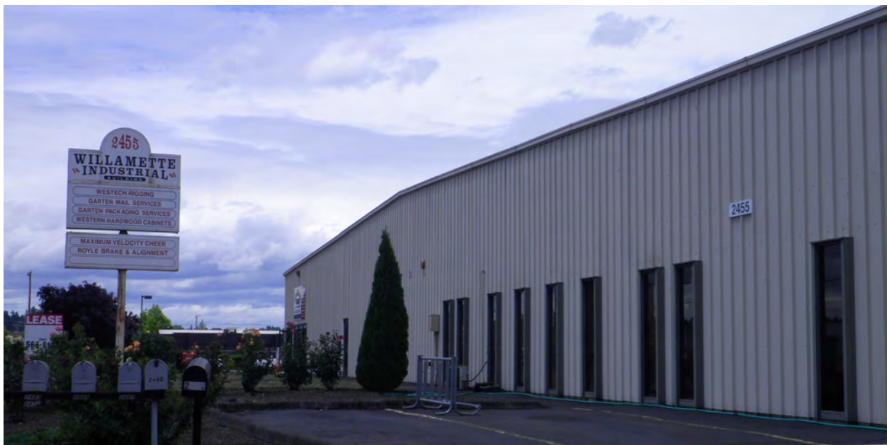
Figure 36 Industrial building in the McGilchrist Street area
