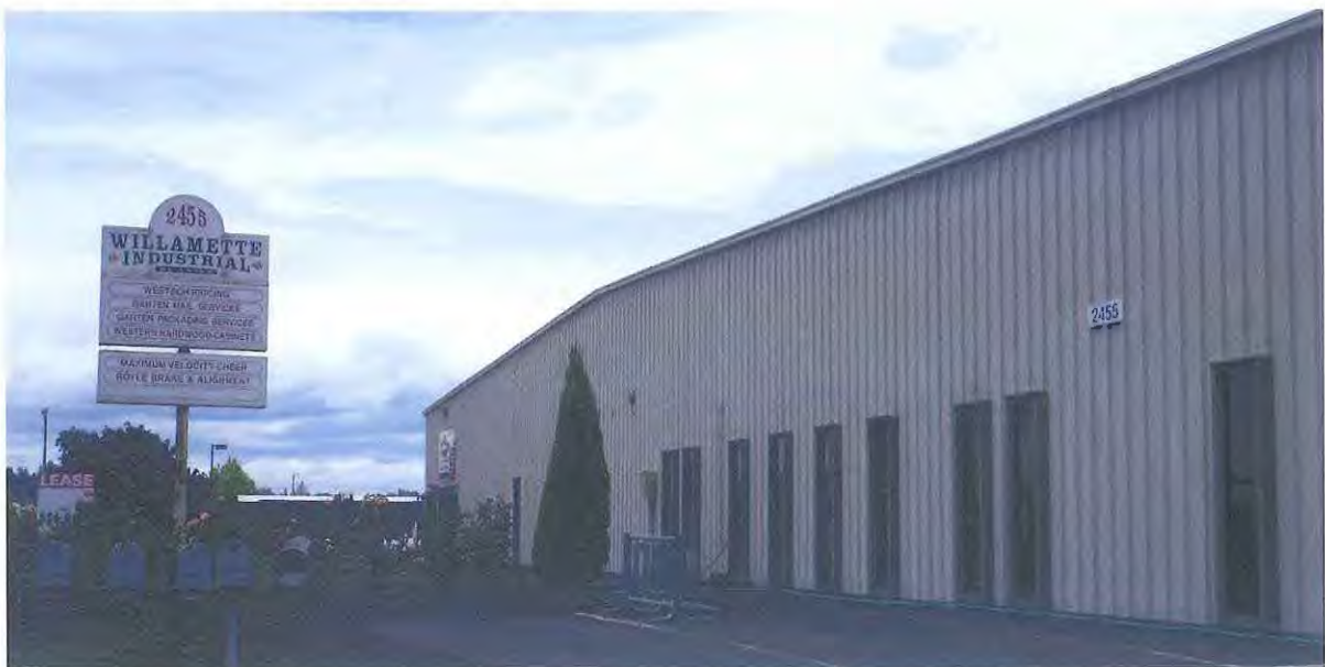
Figure 36 Industrial building in the McGilchrist Street area
