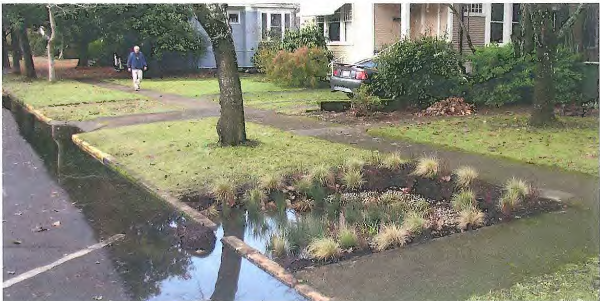
Figure 25 Bioswale on Court Street NE
