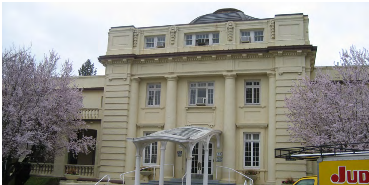
Figure 38 Historic Dome Building
