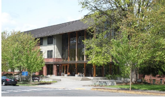
Figure 3.20: Gilbert Hall Exterior
