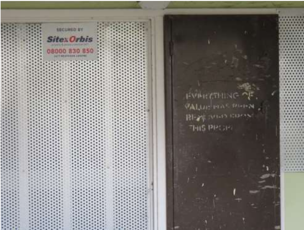
Figure 37. Sheet metal and heavy doors cover entries to empty apartments at Park Hill. Photo: Mackenzie Karp
