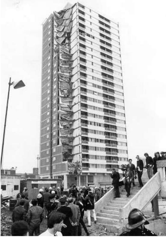
Figure 8. Ronan Point high-rise after 1968 collapse. Source: http://en.wikipedia.org/wiki/Ronan_Point .
