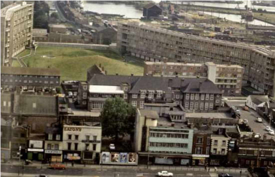
Figure 57. Aerial view of Robin Hood Gardens with central mound. Photo: Alison and Peter Smithson, reproduced in Robin Hood Gardens: Re-Visions . London: RIBA, 2009.
