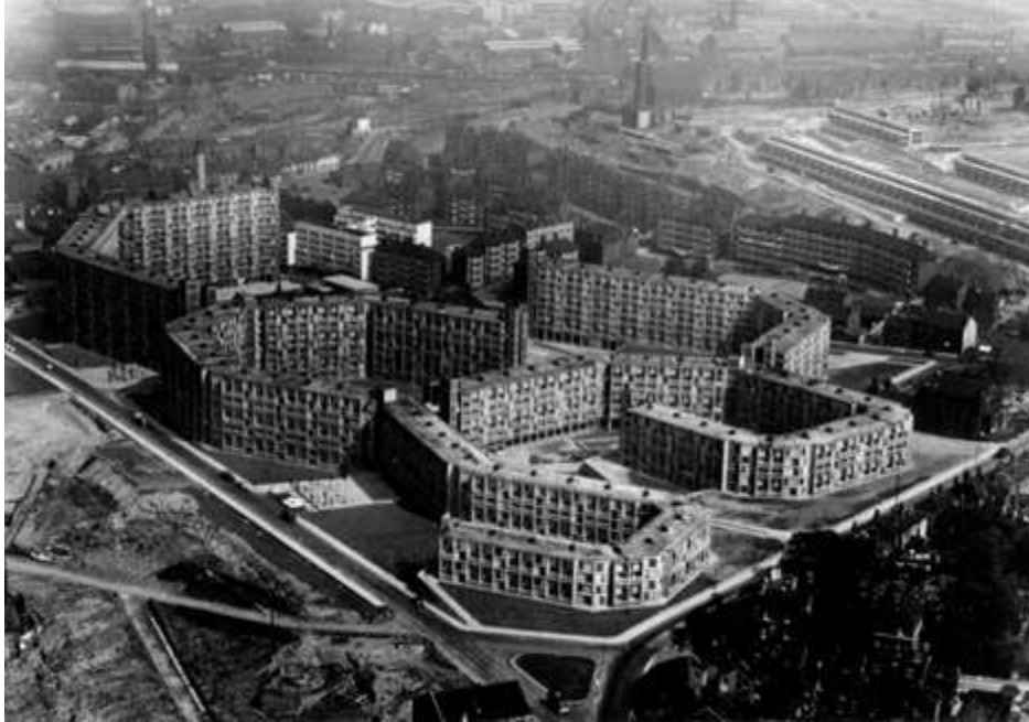
Figure 29. Aerial view of Park Hill, 1962. Source: David Levitt, The Housing Design Handbook , New York: Routledge, 2010.
