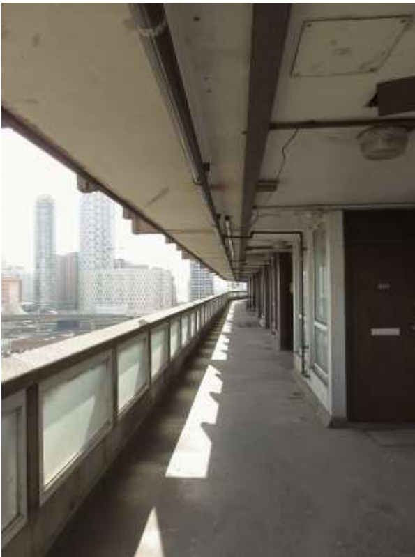
Figure 26. View from access deck of east block of Robin Hood Gardens.
