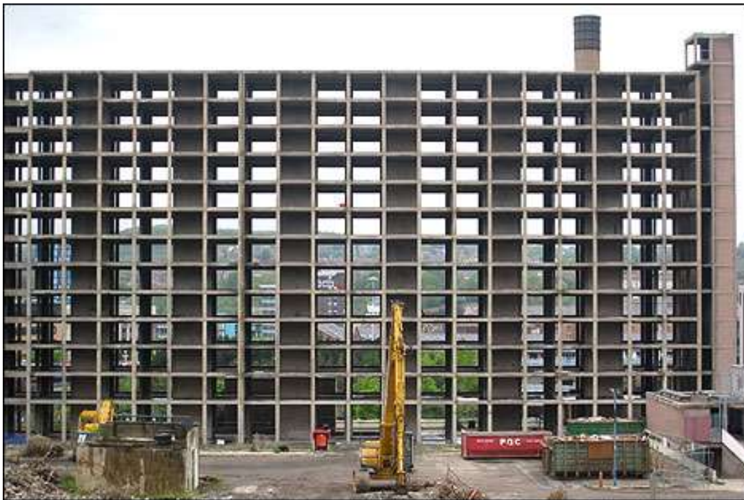
Figure 32. Park Hill stripped to its structural shell. Source: David Levitt, The Housing Design Handbook , New York: Routledge, 2010.
