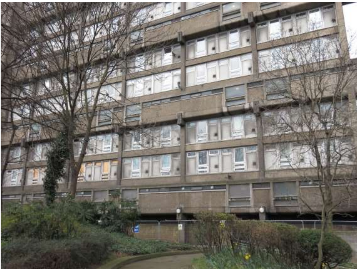
Figure 46. Fencing with “keep out” signs posted around Balfour Tower.
