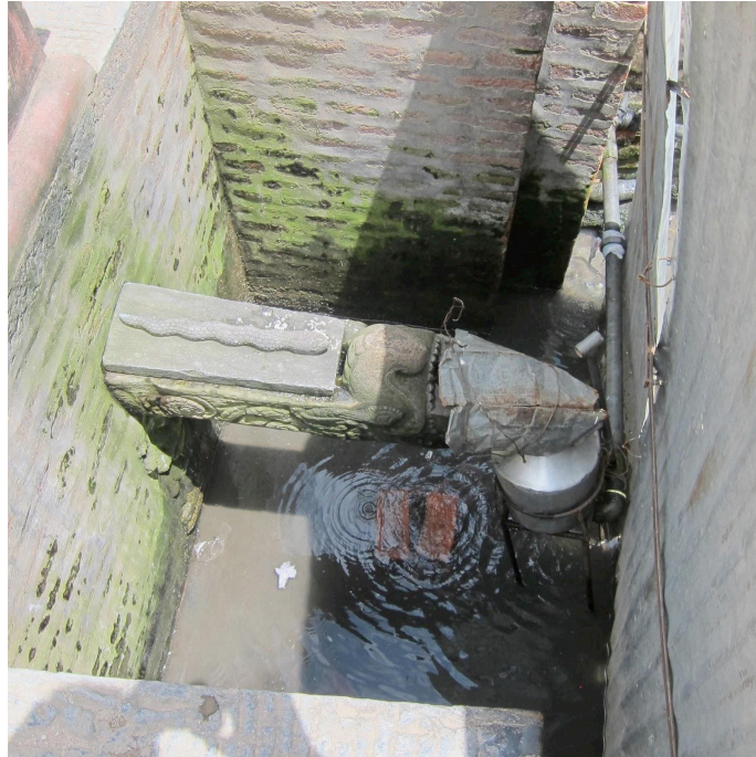
Figure 9: For several hours a day water is diverted away from Washa Hiti to the community reservoir.
