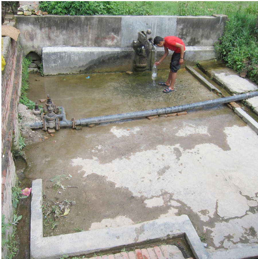
Figure 11: A re-appropriated spout channeling canal water in Harisiddhi, the pipeline cutting through is the metered government pipeline.
