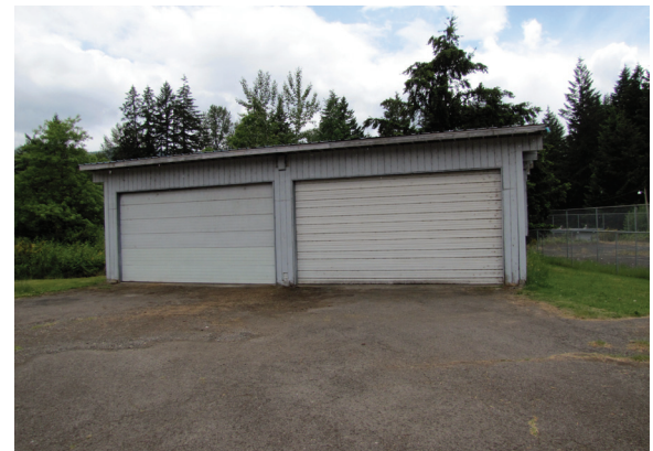
Figure 5.4. Accessory garage building
