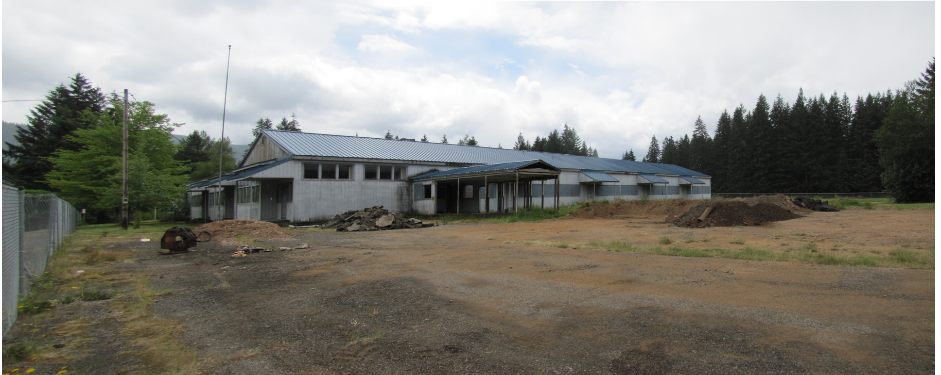
Figure 1. View of existing site
