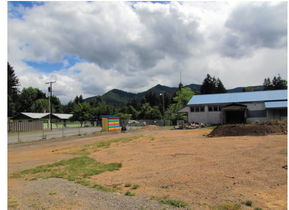
Figure 5.3. View to the SE of the site
