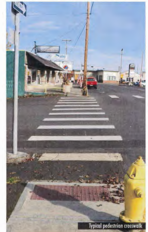
Typical roadway conditions
