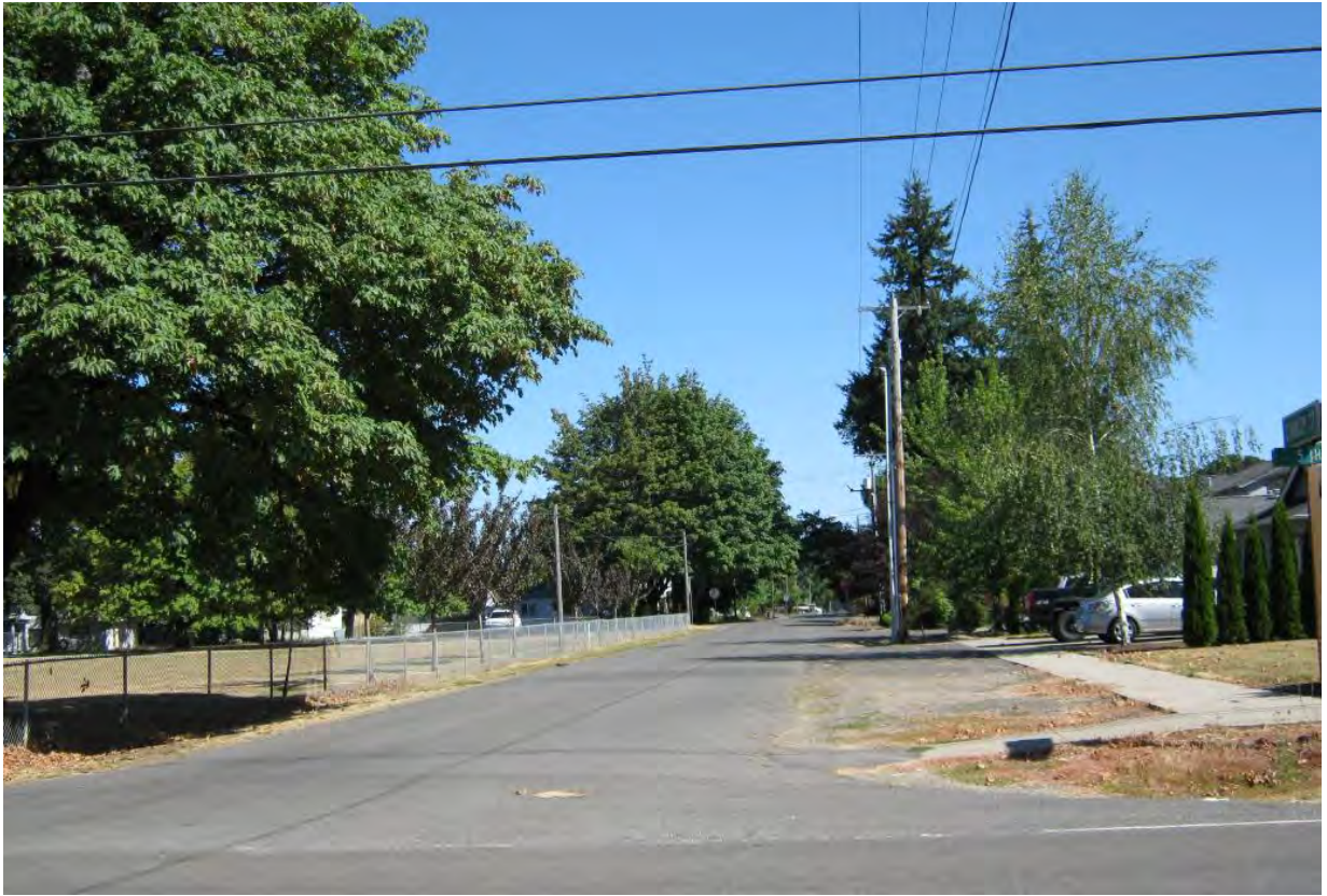
Stanley Street, looking north from OR 153 /5 th Street. The City Park is on the left.
