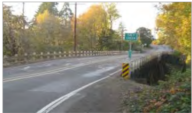
Salt Creek Bridge, looking to the west
