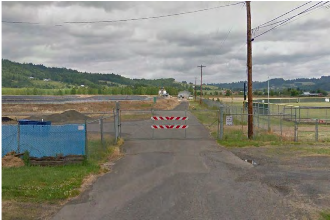
East end of 3 rd Ave, near the new wastewater treatment ponds.
