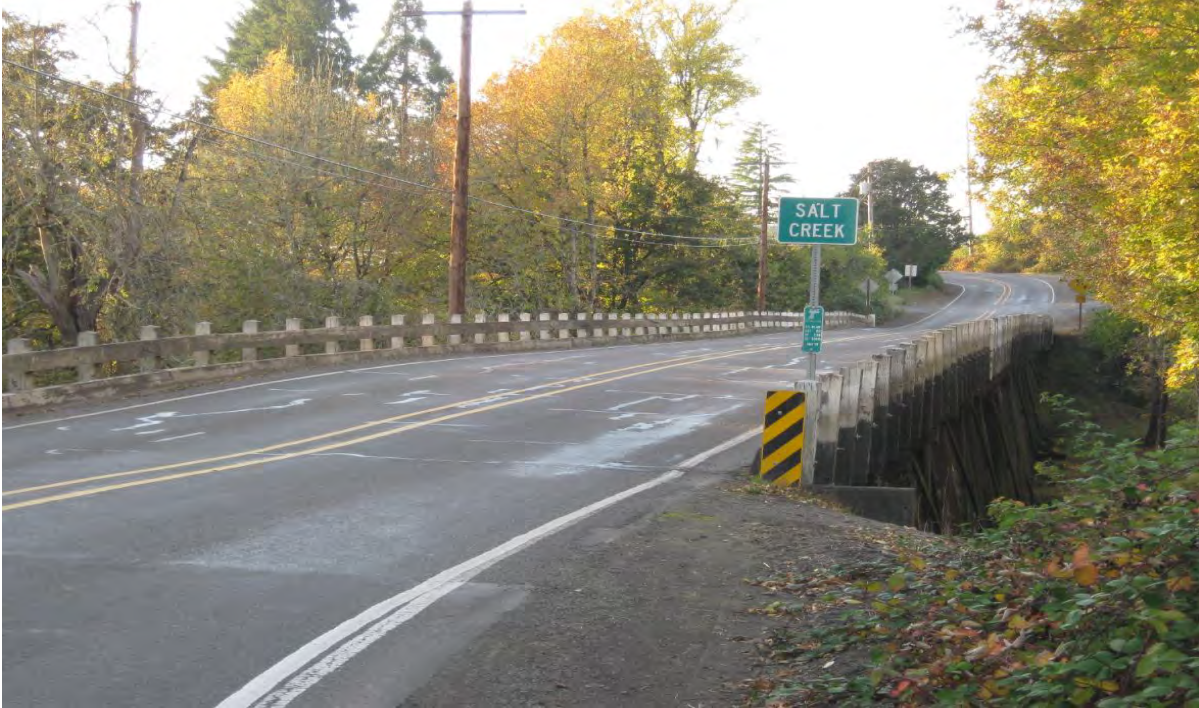
Salt Creek Bridge, looking to the west.
