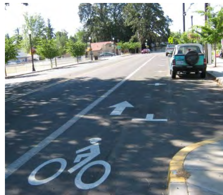
Figure 3 Recent improvements on Trade Street/OR 99W include new sidewalks, bike lanes, and street trees.
