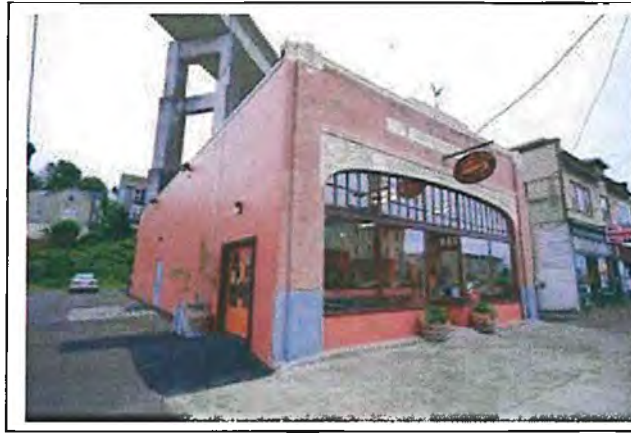
Figure 14.115-5: Non-Industrial Building, Flat Roof Behind Parapet Wall
