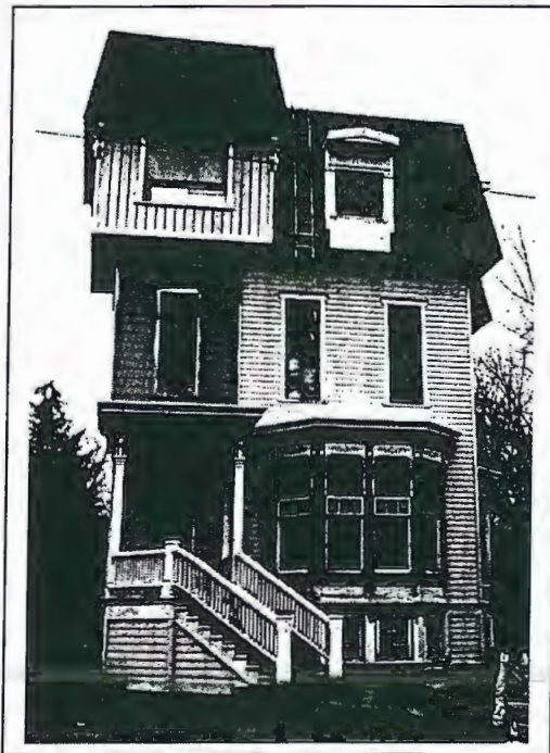
False mansard roof
