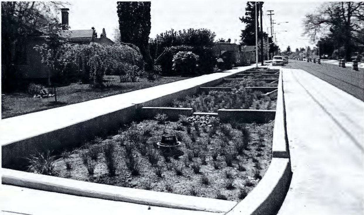
Green street improvement in the Cully Boulevard north area, completed 2011
