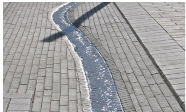
4.7 Engaging rainwater runnel jmlwaterfeaturedesign.com
