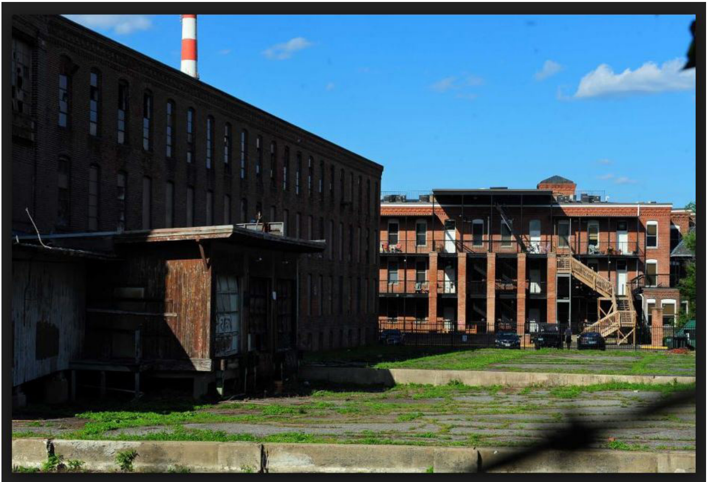
Fig 1.2 Abandoned brownfield next to a housing project, Connecticut
