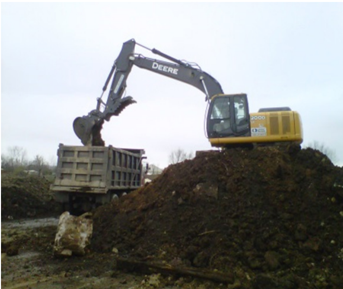
Fig 2.3 Brownfield soil removal
