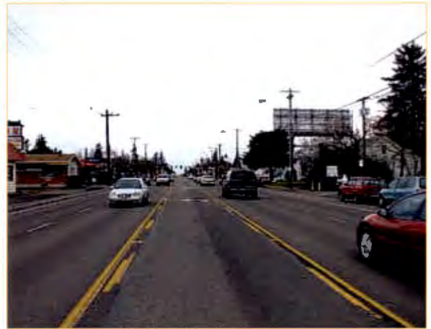
Traffic on SE 122nd Avenue
