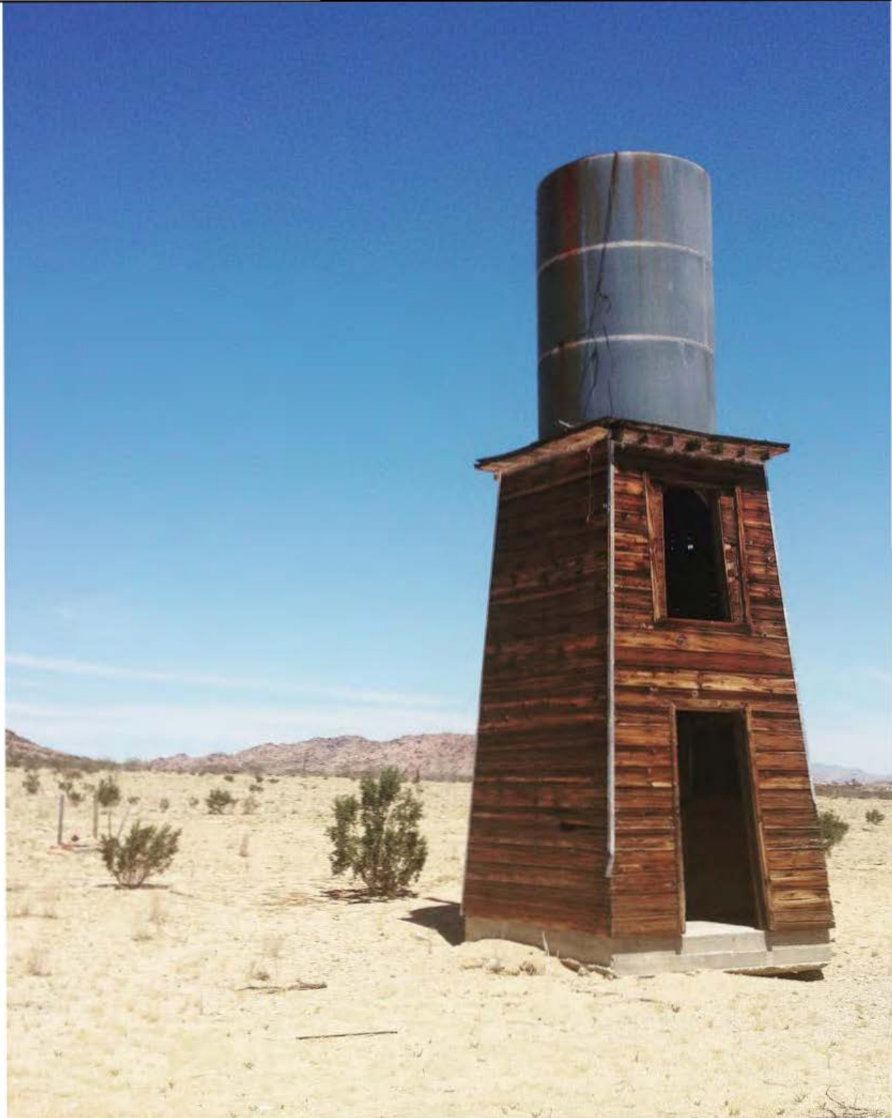
Old water tower. Joshua Tree, CA
