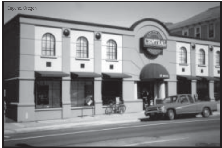
A recent facade upgrade of an older retail building.
