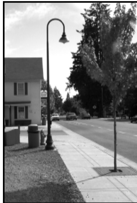
Lighting fixtures downtown should be consistent with the existing lighting theme.
