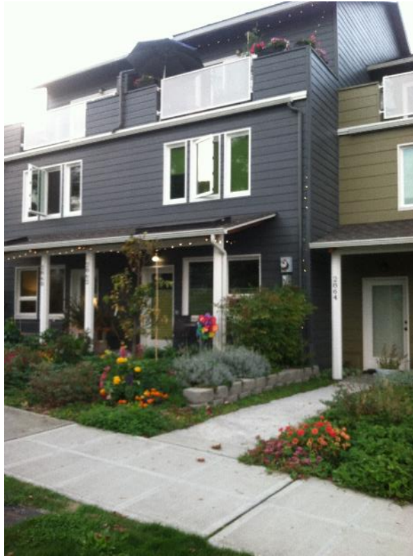
Figure 36: Balconies at for-sale residences north of Central Park
