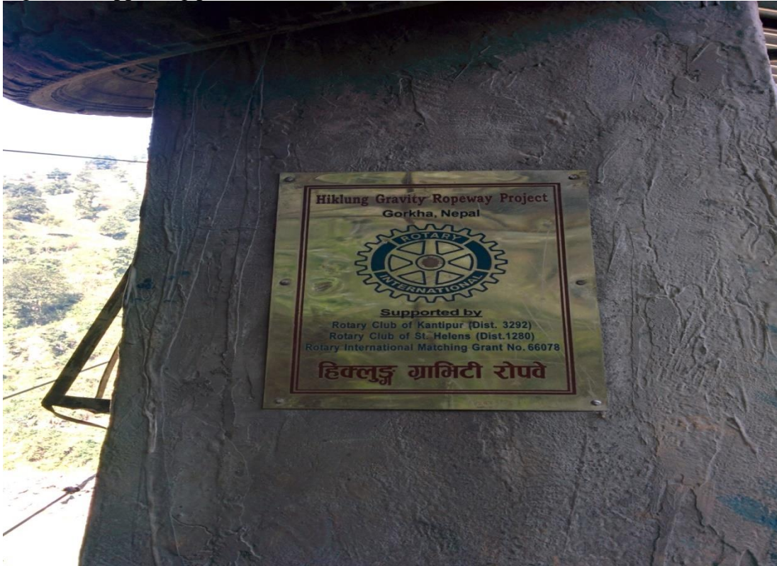
Figure 8. Supporting pillar with name board
