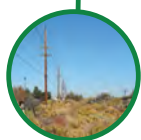
high-voltage power lines run next to the railroad tracks
