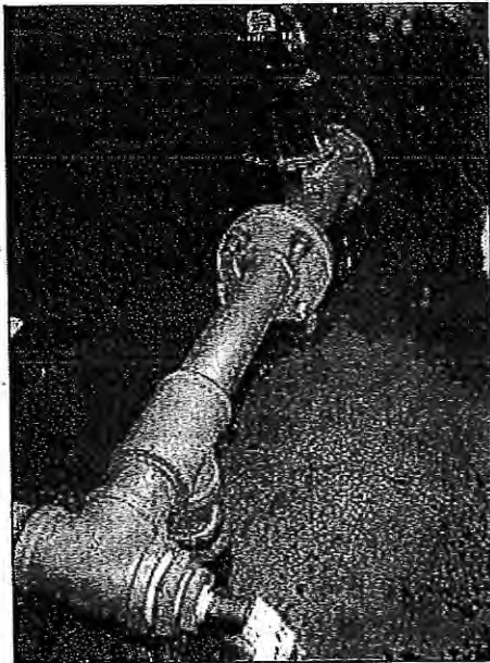
Well #1 Flow Meter
