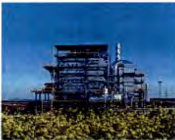
Biomass Plant From: Gestamp
