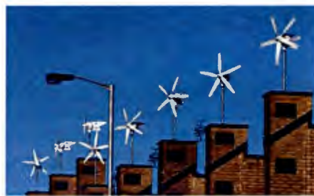
Small-scale wind turbines mounted on a roof.
