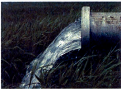
In-Outfall Pipe Micro-Hydro System
