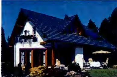
Roof-top solar panels on a single-family residence.
