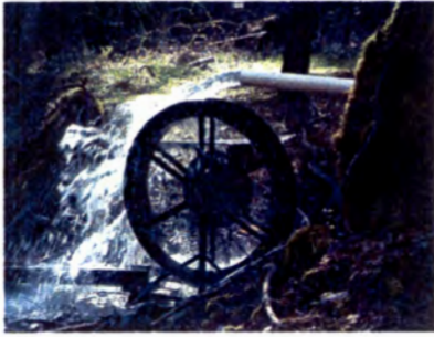
In-stream Micro-Hydro System
