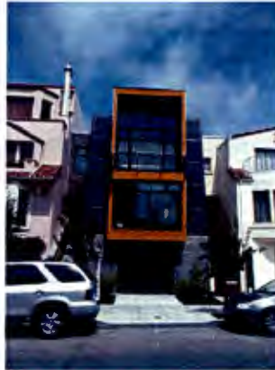
Integrated solar wall panels on a townhouse.
