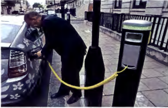
Single Electric Vehicle Charging Station on Street
