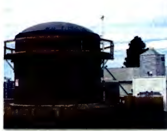
Biogas/Methane Production Facility
