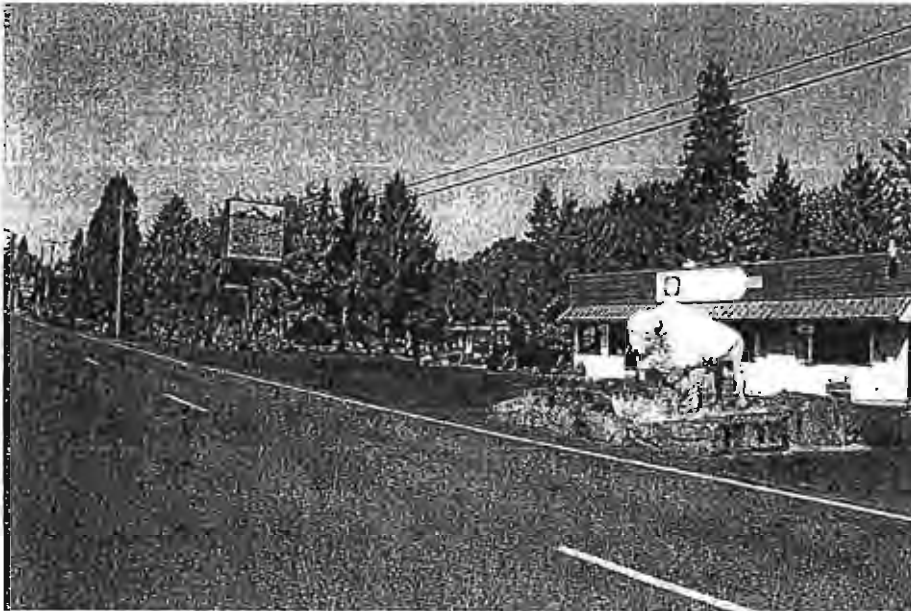
View looking west along Westcliff Drive showing the White Buffalo building and the Vagabond Lodge sign. The extent of the Vagabond Lodge property frontage extends from the near power pole to the next power pole
