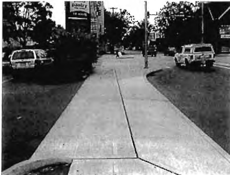
Top: Decorative residential driveway apron with set pavers Bottom: Commercial driveway apron with sidewalk
