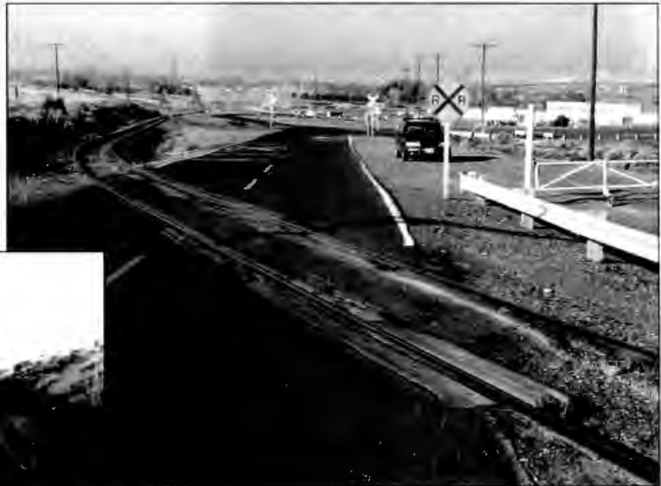
Angled railroad crossing with damaged flangeways on Devore Road at base of hill.
