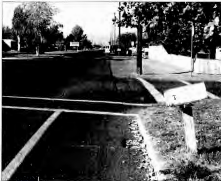
Bike lane on Columbia Street is dropped a block before the school
