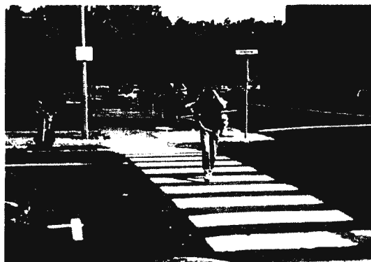
Zebra crosswalks are more visible to drivers than standard double lines.
