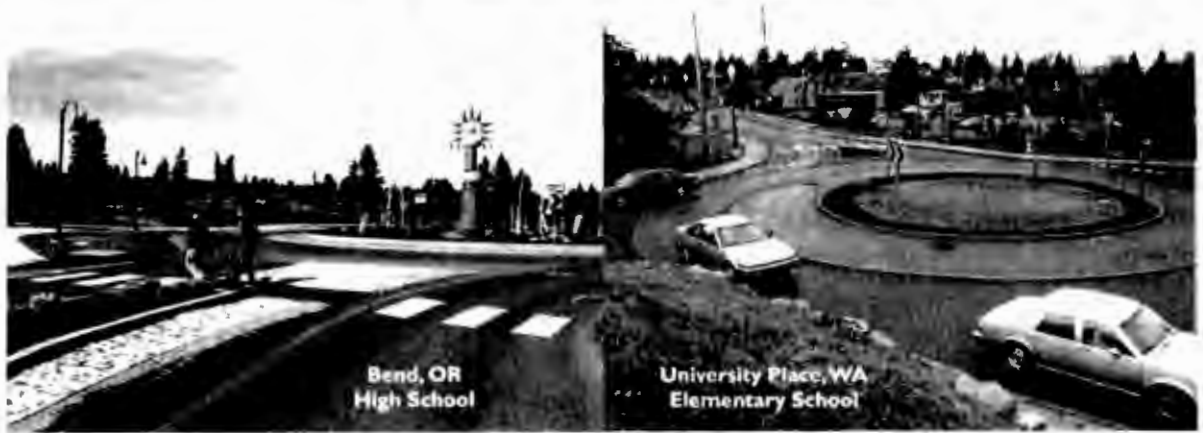
Figure 12.4-8 School Access Using a Roundabout
