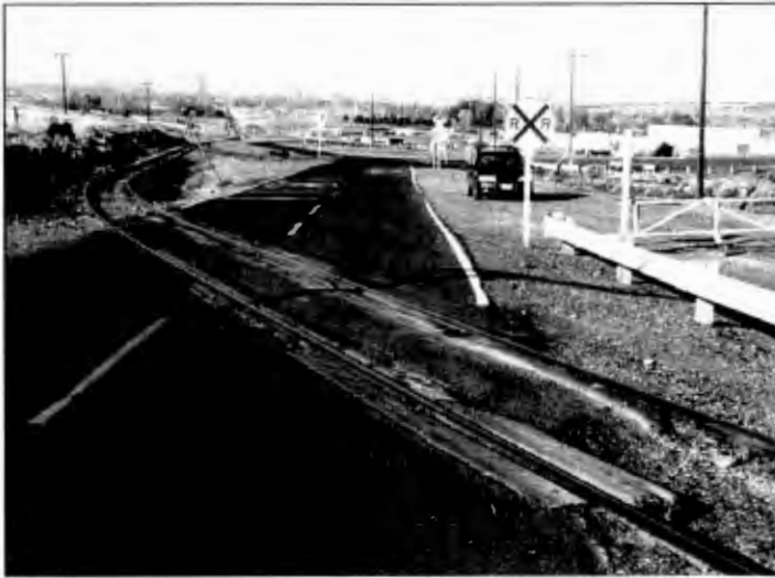
Angled tracks with a rough irregular flange opening can easily cause a cyclist to fall
