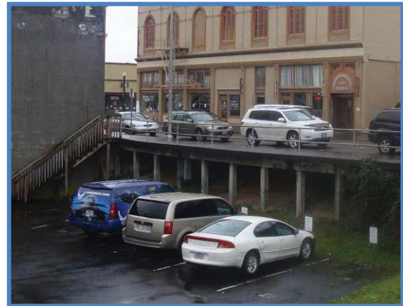
Exposed Chair-wall System at 10 th and Duane
