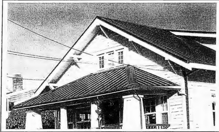
High profile metal seam roof
