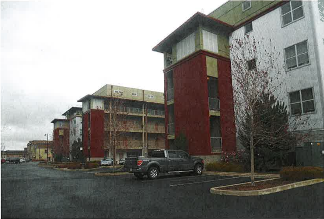
Cannery Loft Condominiums; ground floor industrial/limited commercial units with residential units above
