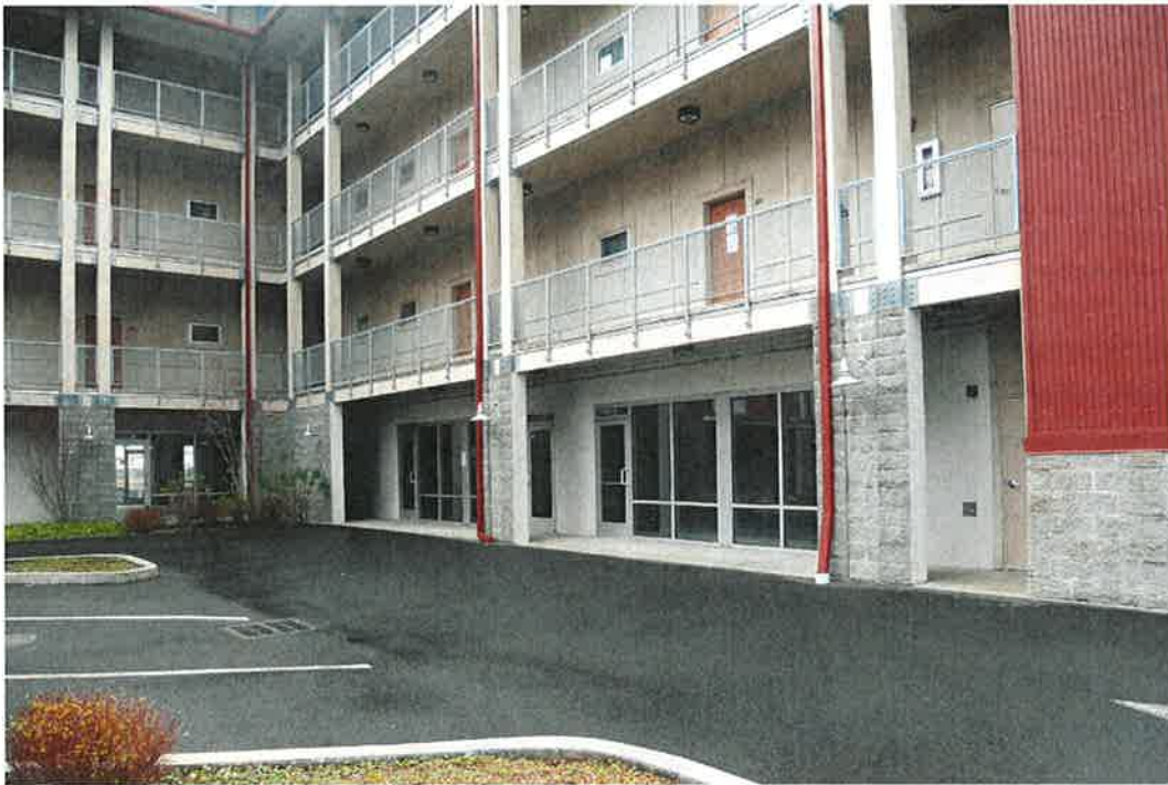
Typical industrial/limited commercial unit
