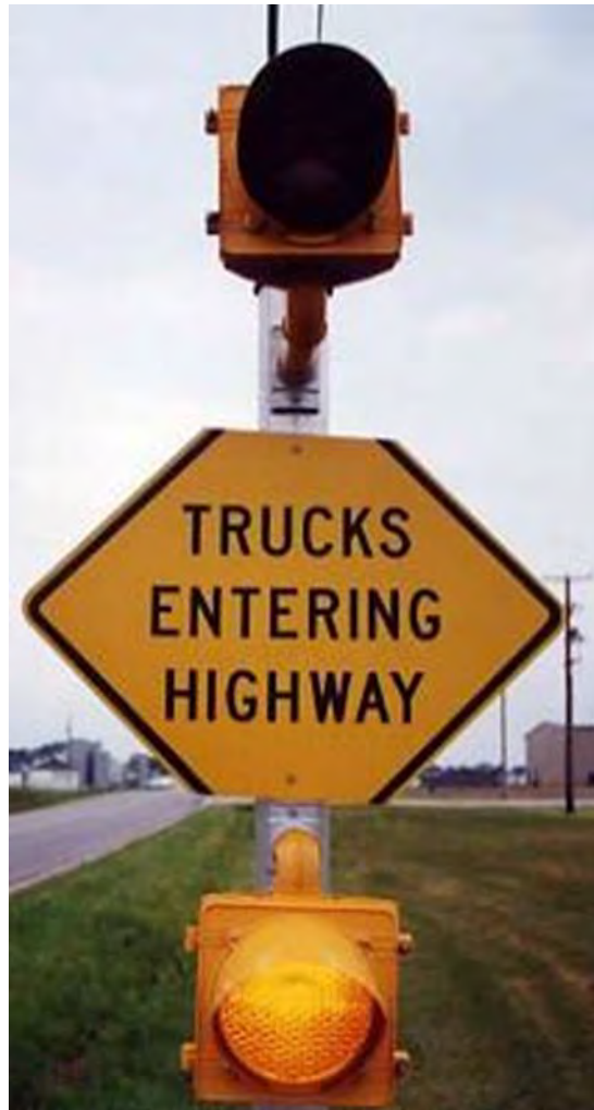
Figure 5-5: Supplemental flashing beacons.
