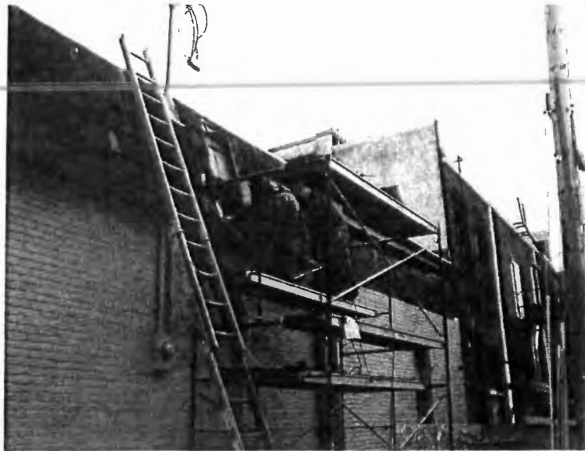
Ongoing restoration of 501 E. Main Street, funded through Historic Renovation Grant program, 2010.
