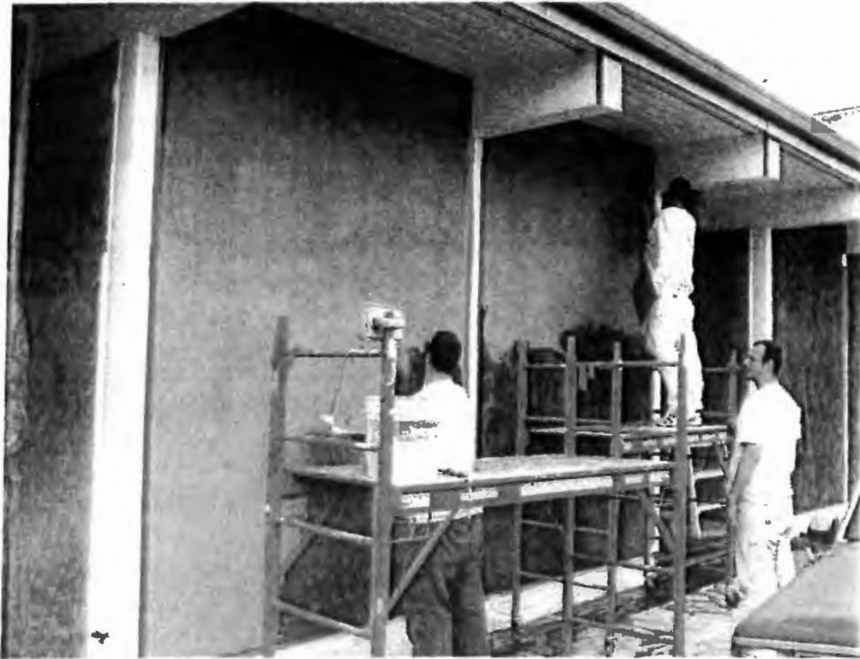
Ongoing restoration of 802 E. Main Street, funded through Historic Renovation Grant program, 2012.
