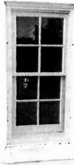
Restored window at the Cottage Grove Armory.
