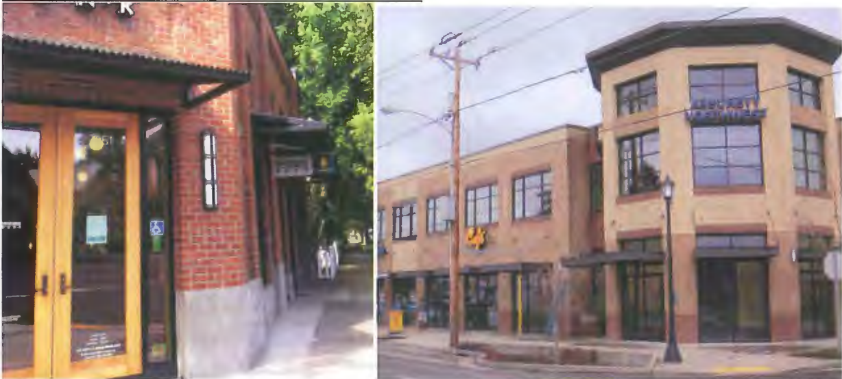
Figure 14: Examples of awnings over all windows and doors
