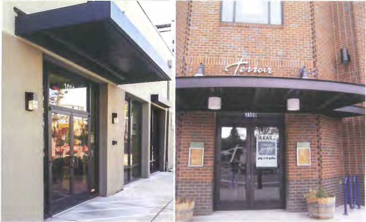
Figure 13: Examples of awnings over building entrance
