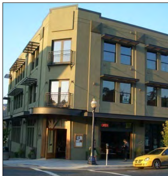
FIGURE 531-23 PRIMARY BUILDING ENTRY LOCATED AT CHAMFERED BUILDING CORNER
