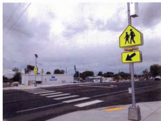
Exhibit 2 – Example of an RRFB (Irrigon, OR)
