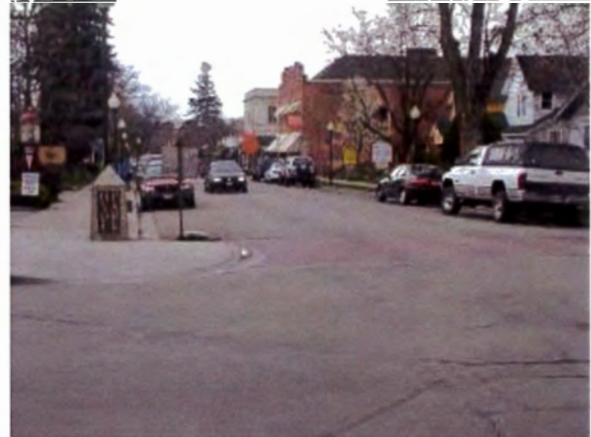
Exhibit 3 – Example of a Curb Extension (Boise, ID)
