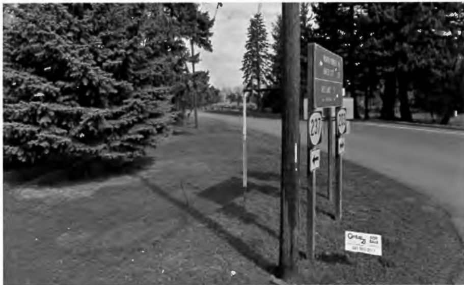
Exhibit 2A Limited Intersection Sight Distance at the OR 203/Bryan Street Intersection; from Bryan Street EB viewing north (top)
