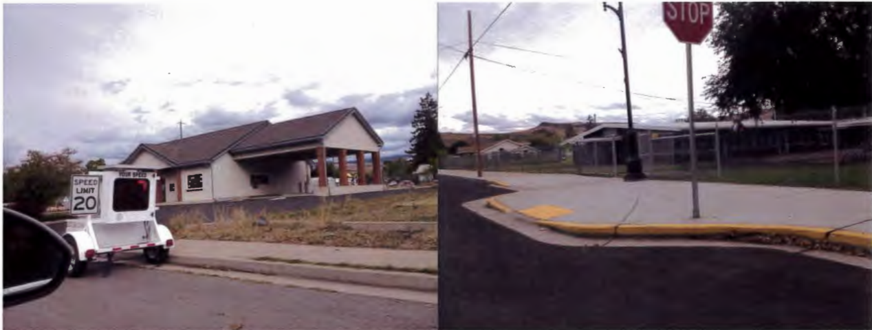
Exhibit 7 Speed reader board (left) and curb extension (right), both located near Union schools.
