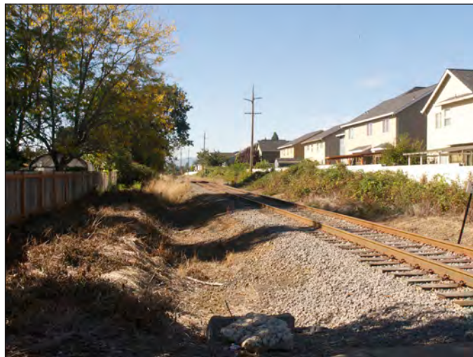
Rail corridor through Cornelius
