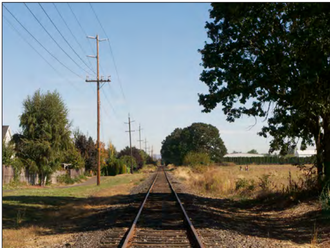
Rail corridor through Cornelius
