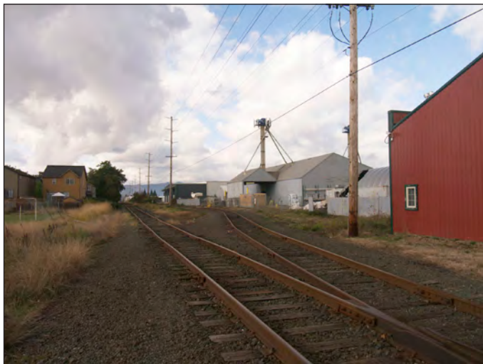
Rail siding west of N 10th Ave.
