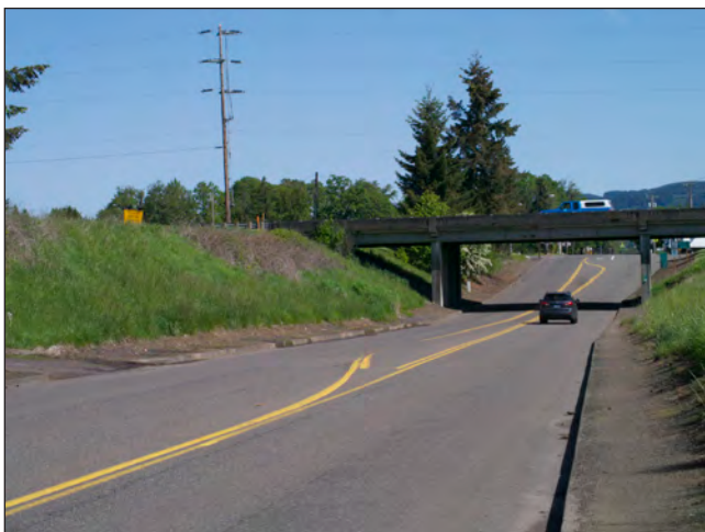
Oregon 6/Oregon 47 undercrossing looking south
