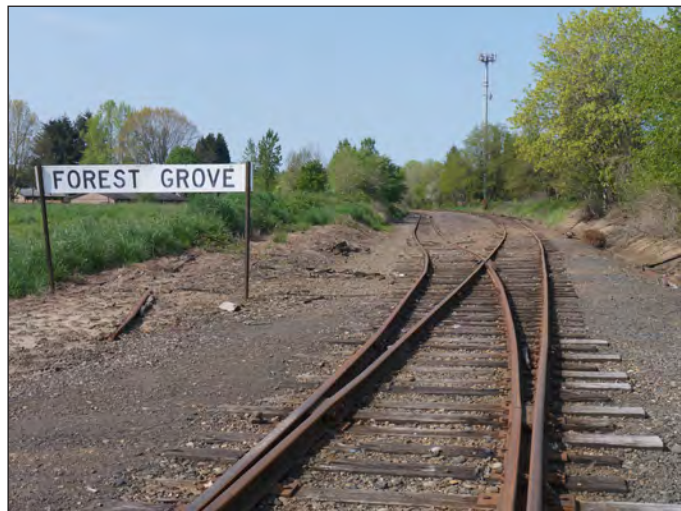
Rail corridor near Hawthorne Street
