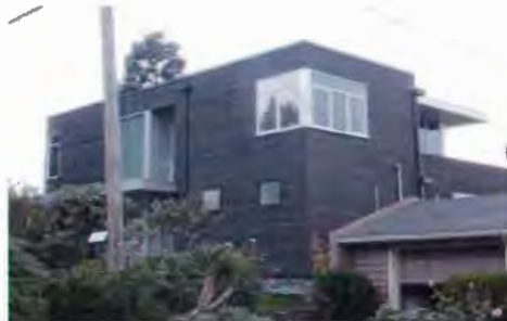
An Example of New Construction With Inappropriate Materials and Finishes
