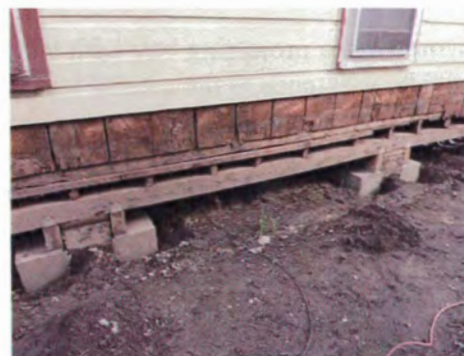
Example of an Inexpensive Brick Pier Reinforcement to be Covered With Wood Skirting on Completion
