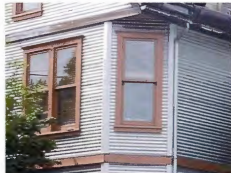
Well-Crafted Matching Wood Window Replacement Inappropriate Siding and Trim Replacement
