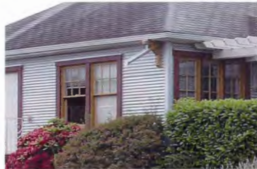
Example of an Inappropriate Siding Revision
