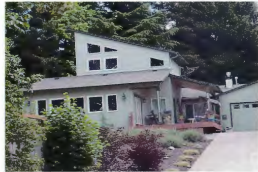
Example of a Historically Inappropriately-Shaped Building, Roof and Windows
