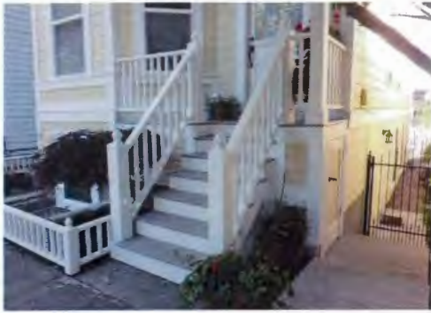
Example of a Single-Story Cottage Raised 3 Feet to Allow Lower Level Improvements; the Historic Relationship to the Ground is Retained
