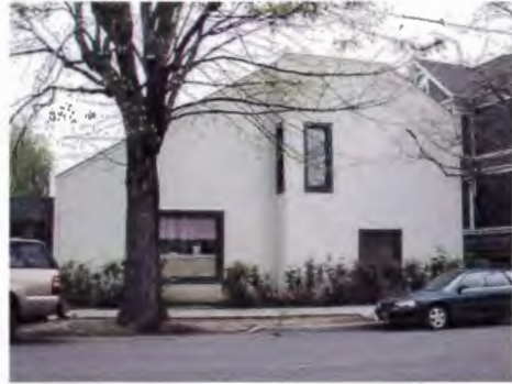
Example of a Non-Complying Roof Shape, General Lack of Trim and Type of Siding
