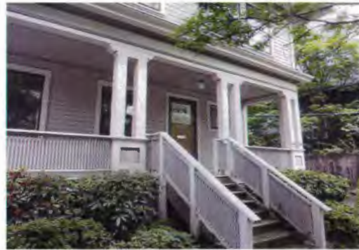
Example of a Front Porch and Stair Appropriately Modified to Meet Current Building Codes For Handrails
