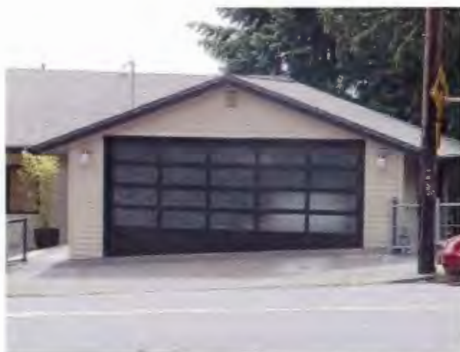
An Inappropriate Mostly Glass Garage Door
