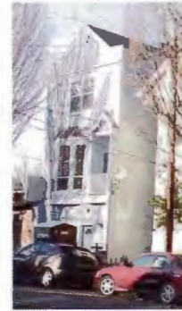
Example of a Single-Story Cottage Turned into a Tall, Skinny Structure Resulting in the Loss of its Historic Relationship to the Ground
