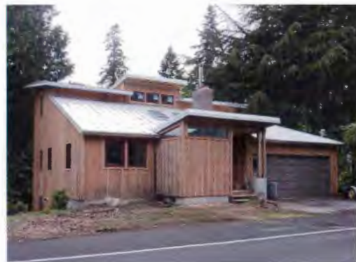
Example of Non-Complying Shed Roof Shapes, and Sheet Metal Roofing Materials
