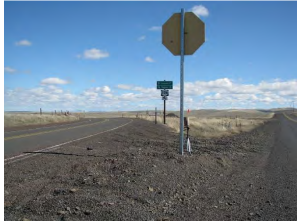
Exhibit 6-2. Restricted Sight Distance at OR 206/Lonerock Road
