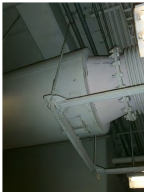
Figure 11 .Silencer without lateral bracing
