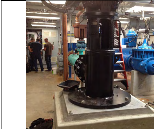
New backwash pump installed in 2012.
