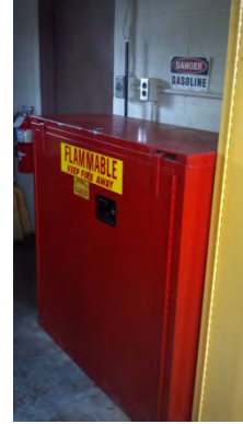
Figure 2. Hazardous Material cabinet is not anchored.
