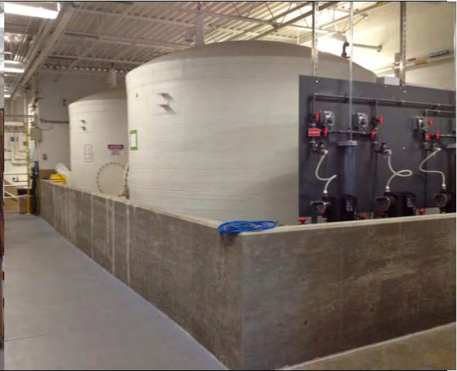
Coagulant storage with containment area and metering pumps. Tanks cannot be removed or replaced without significant effort.
