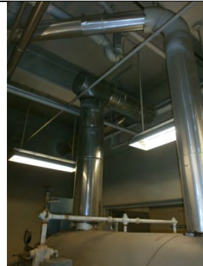
Figure 16. Hot Water pipes are not braced laterally.
