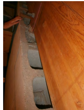
Figure 34. Penthouse crawlspace: The masonry blocks are not fully grouted
