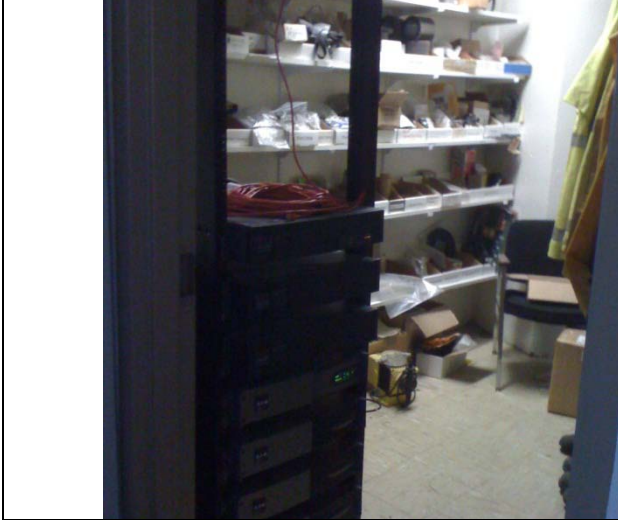
Portion of server room used for storage.
