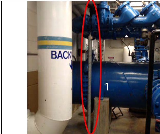
1. Pipe support not adequate for seismic event.
