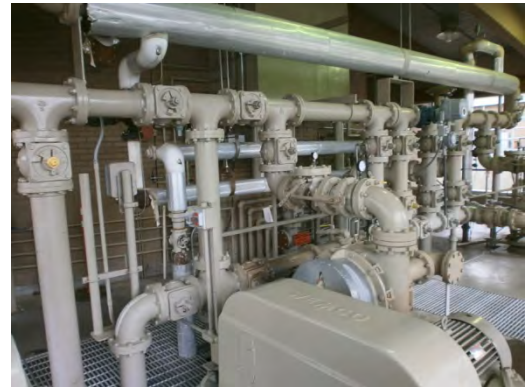
Figure 4. Piping in Digester Control Building requires bracing
