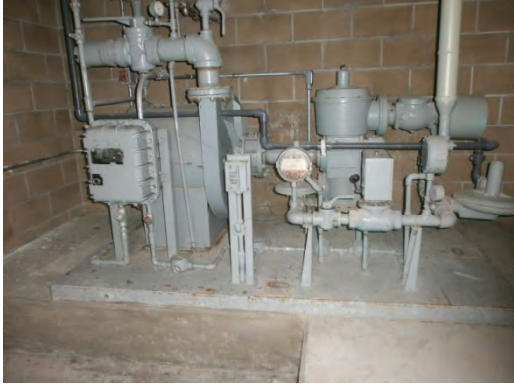
Figure 7. Pump Skid outside of the Digester Control Building is not anchored
