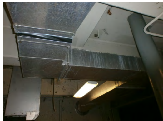
Figure 24. Duct work requires bracing
