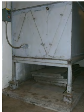
Figure 6. Blower unit is not anchored properly
