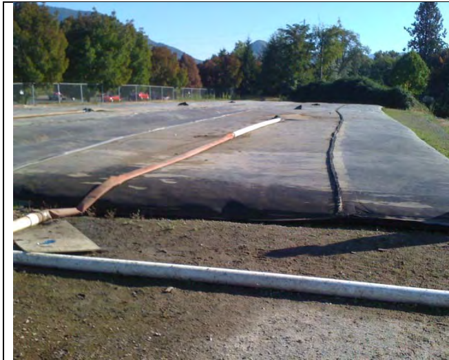
Geobags in use at Mill Pond.
