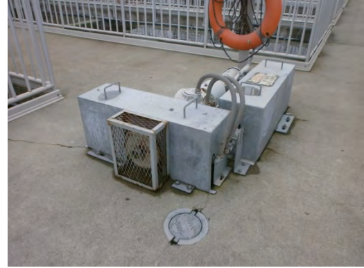
Figure 2. Cracks in the elevated deck were observed at the openings.
