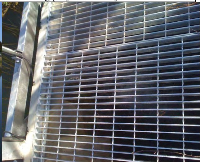
Effluent gate to Skunk Creek.
