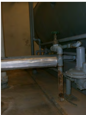
Figure 17. Deterioration of a pipe support in the boiler room
