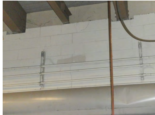
Figure 22. Diagonal Cracking in the West wall of the workshop due to settlement
