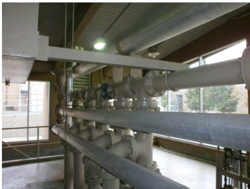
Figure 5. Piping in Digester Control Building requires bracing
