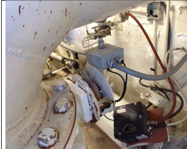
Maintenance made challenging by space constraints.
