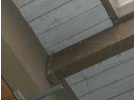
Figure 25. Reinforcement of the deck at the diaphragm performed with joist hangers without provisions for lateral loads
