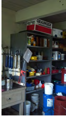
Figure 1. Unanchored storage rack
