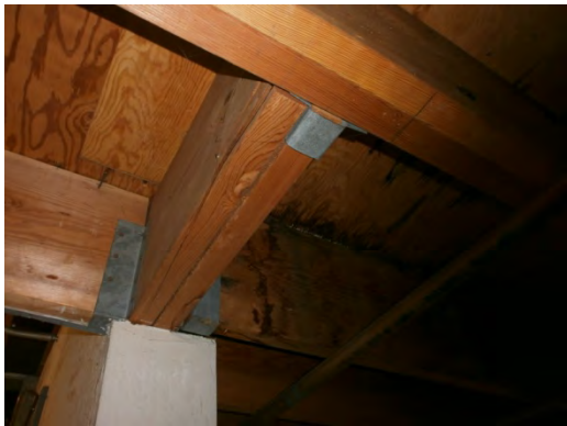
Figure 33. Joist connections do not have positive capacity for diaphragm shear in the penthouse roof deck.
