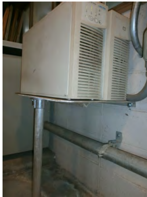
Figure 3. UPS batteries are resting on a shelf without any restraint against lateral movements
