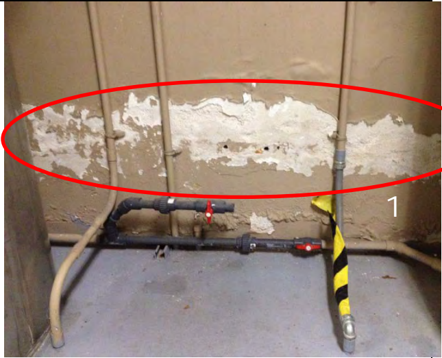
1. Paint failure.
