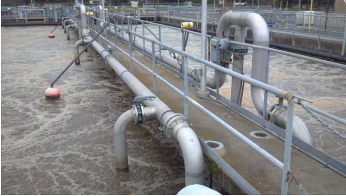
Figure 1. Air piping has long unsupported vertical runs in the Aeration Basins
