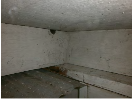
Figure 1. No positive connection between the roof diaphragm and top of shear wall
