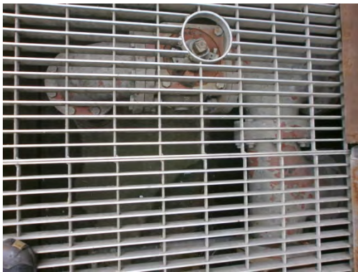
Figure 3. Failure of coating of the piping
