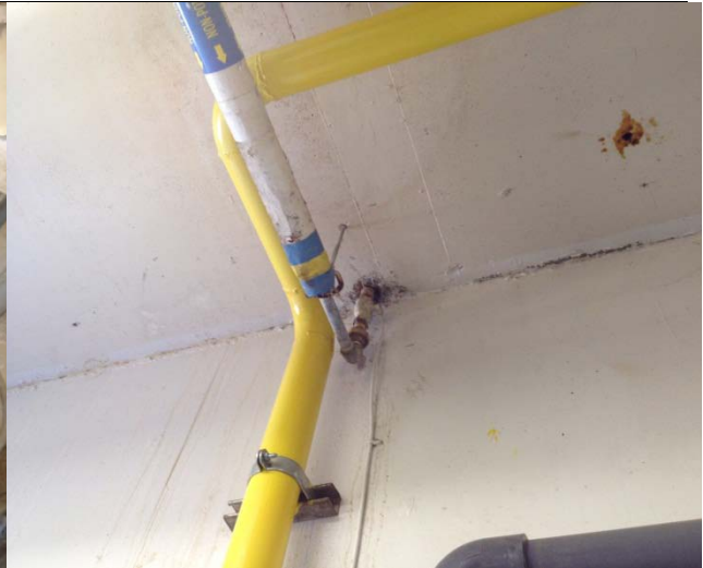
Piping is not seismically supported.
