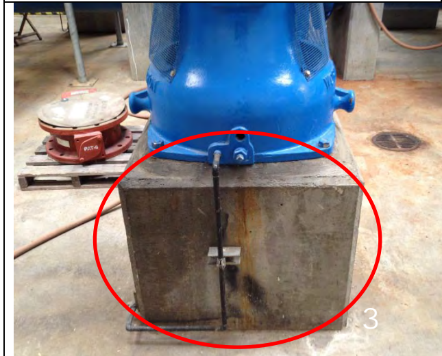
3. Pad not adequately sized for seismic event.
