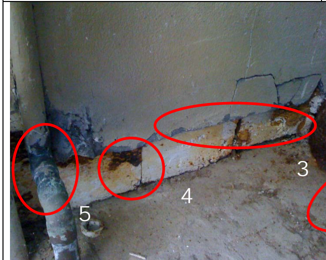
3. Paint deterioration. 4. CMU deterioration. 5. Pipe coating corrosion.
