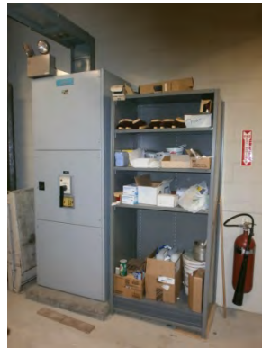
Figure 40. Storage racks and electrical cabinets are not anchored properly
