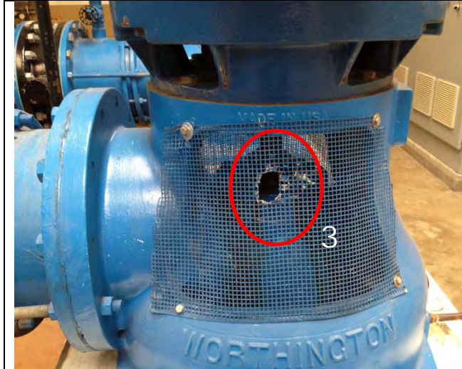
3. Damage to screen poses a potential safety concern.
