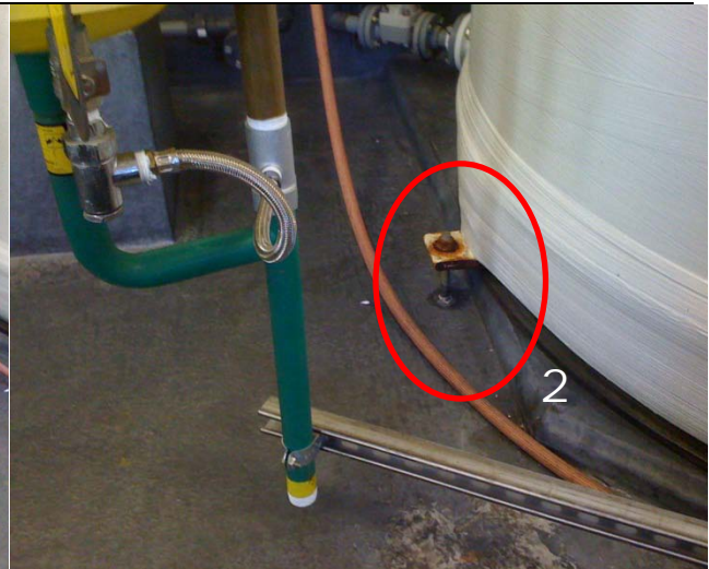
2. Tanks may not be adequately anchored for seismic event. Corrosion observed on existing anchors.
