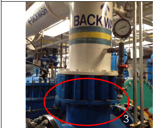
3. Valve may be failing. Difficult access and location for replacement and maintenance activities.
