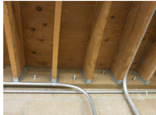
Figure 4. Incorrect detailing at the roof to wall connection of the Headworks electrical building will cause cross grain bending in the ledger block
