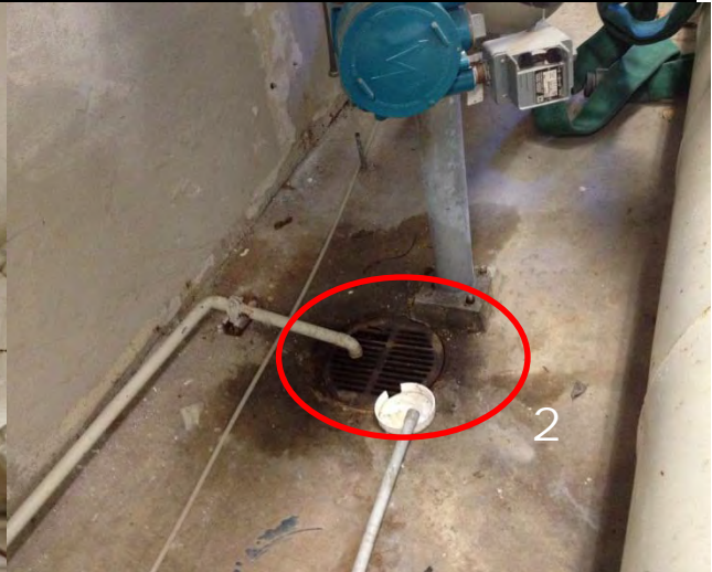
2. Drain line(s) may be undersized to handle major leaks or emergencies.
