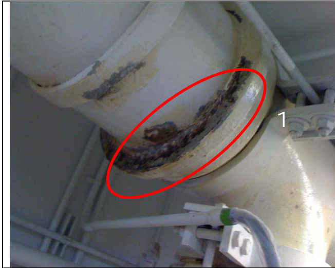
1. Pipe joint corrosion.
