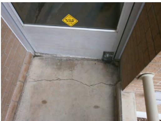
Figure 29. Crack on the concrete elevated slab, outside of the dewatering room entrance.
