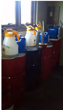
Figure 3. Oil barrels do not have a containment area to protect against spilling. The barrels are not anchored to the walls.
