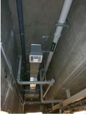
Figure 7. Duct work in the basement of the Headworks Electrical Building requires additional bracing
