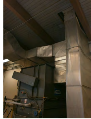
Figure 26. Long tall vertical duct work without bracing
