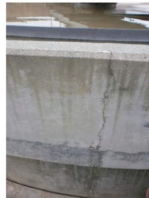
Figure 4. Shrinkage cracks were observed on the tank walls above grade.
