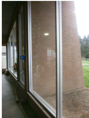
Figure 3. Untempered glass on the south side of the Digester Control Building
