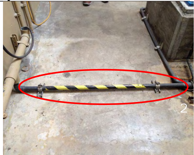
2. Trip hazard identified.
