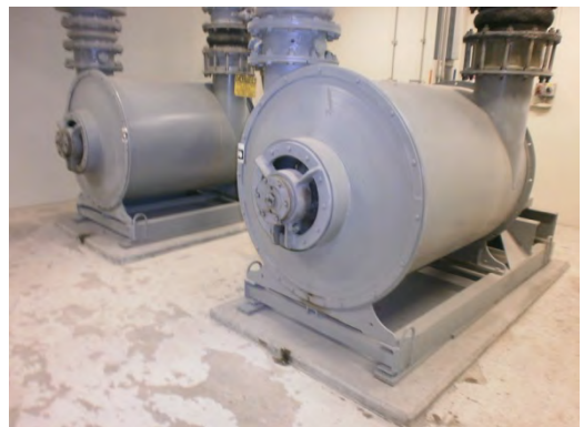
Figure 18. Old blowers are not anchored
