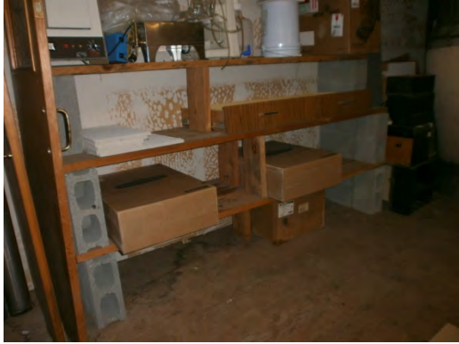
Figure 31. Makeshift Storage rack in the penthouse will be unstable during an earthquake
