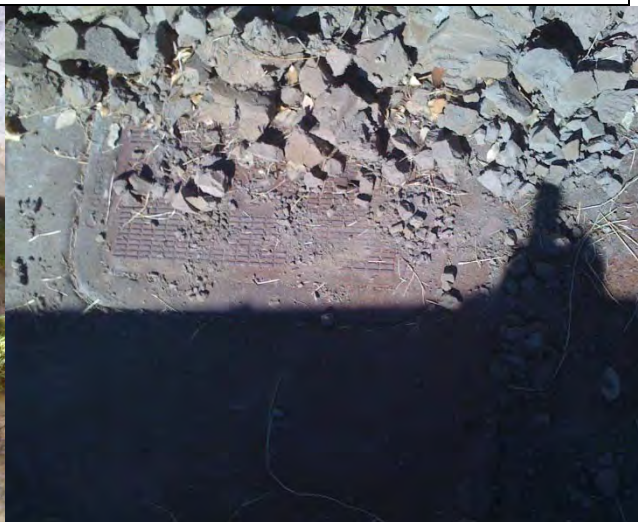
Space constraints on-site can lead to encroachment of access to valve boxes during solids dewatering.
