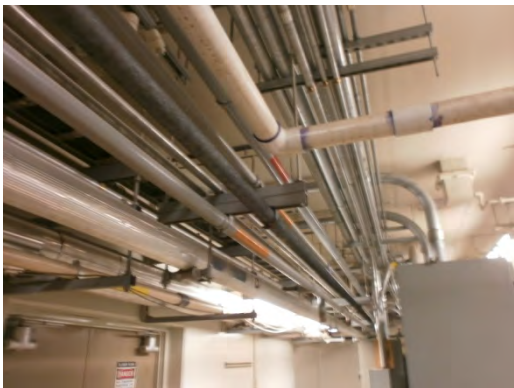
Figure 5. Several suspended pipes including a Natural Gas Pipe are not braced properly against lateral loads.
