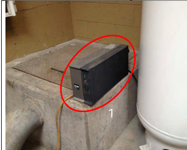
1. Separate housing for battery back-up power supply to protect from potential leaks.
