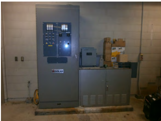
Figure 41. Electrical cabinets are not anchored properly
