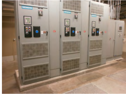
Figure 4. Electrical Cabinets are only anchored on one side.
