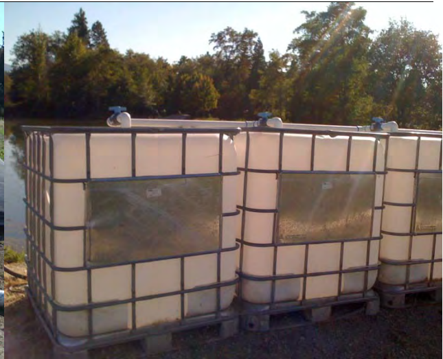
Dewatering polymer feed system.
