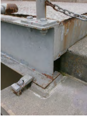
Figure 7. Walkway bridge bearing requires strengthening.
