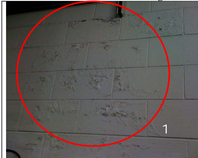
1. Paint failure.
