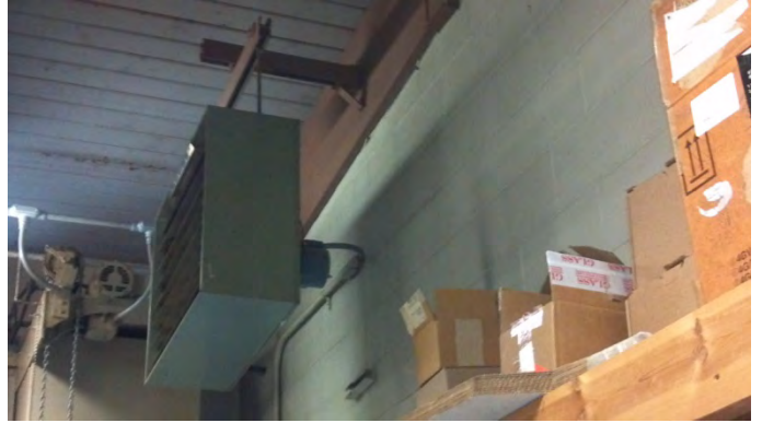
Figure 8 .Heater without side bracing
