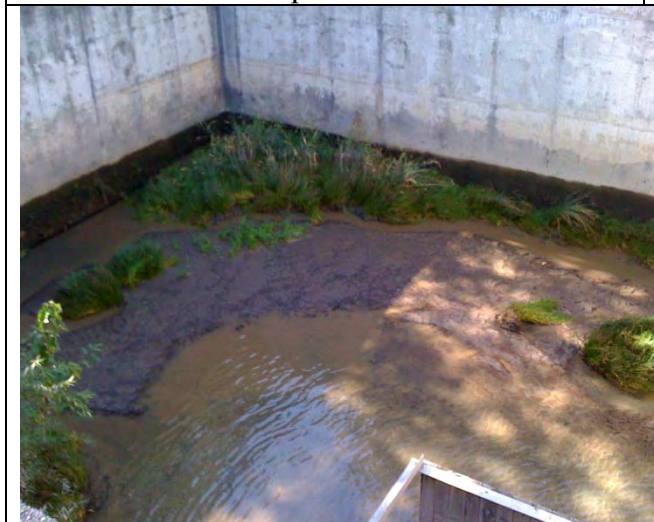
Cleaning and maintenance of washwater equalization basin is extremely labor-intensive because accessing the bottom is difficult. As a result, unwanted vegetation growth is common.
