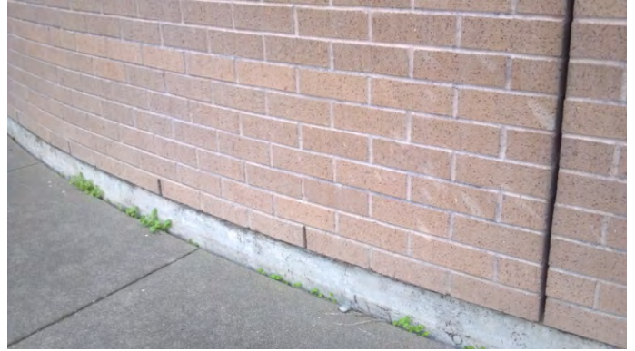
Figure 2. Brick veneer on Digester No.1 is installed with dovetail anchors and weep holes are provided
