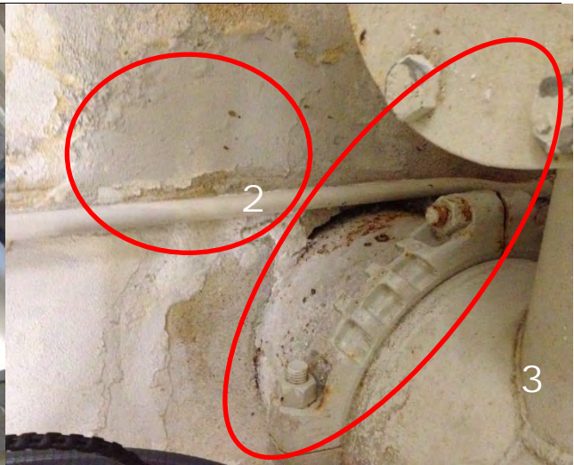
2. Wall cladding and paint deterioration. 3. Corrosion.
