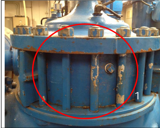
1. Corrosion.
