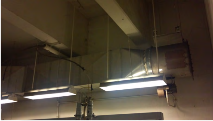
Figure 1. Ductwork Requires Bracing
