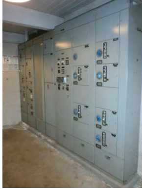
Figure 1. MCC cabinet is anchored to the wall behind using a small clip angle. Signs of moisture penetration through the building wall, is apparent on the concrete pad.
