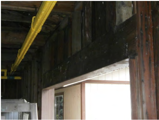
Figure 3. Large opening with a weak collector beam above the opening.
