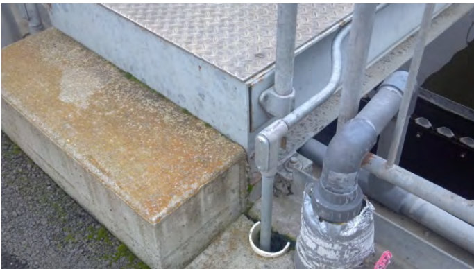
Figure 5. The walkway bridge bearing on the Clarifier wall requires strengthening.
