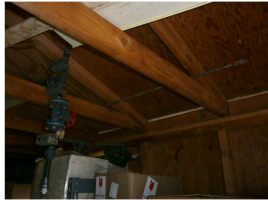
Figure 4. Storage shed has unanchored storage racks and piping
