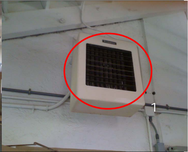
1. Example electric heater used in multiple locations around the plant. The plant lacks an optimized central climate control system.
