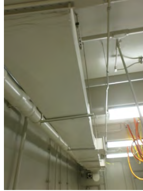
Figure 2. Cable Tray Requires Bracing
