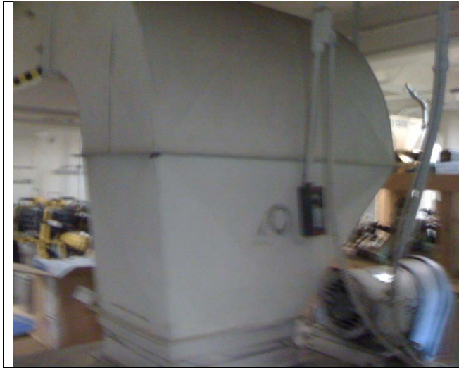
Main duct for air flow to operations building.
