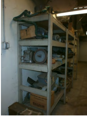
Figure 13. Storage Rack Requires Bracing
