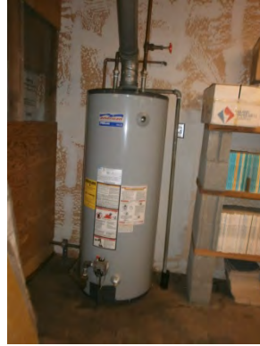
Figure 38. Water heater in the penthouse is not braced properly
