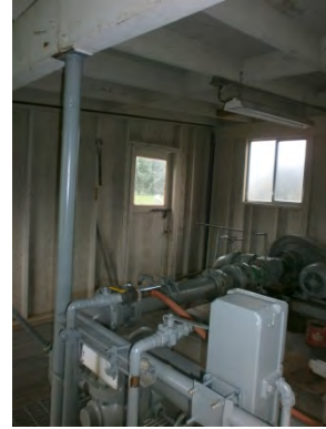
Figure 2. Center columns supporting the roof beams have little to none lateral support capacity
