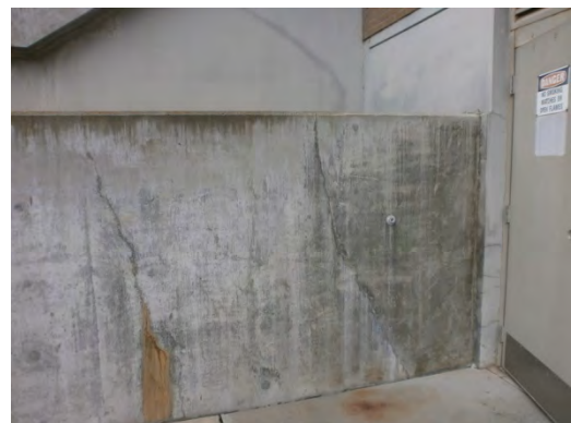
Figure 30. Cracks on the short wall, west of the pump room entrance. It shows the extent of settlement damage
