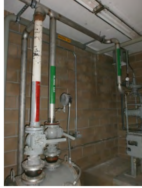
Figure 8. Miscellaneous piping in the Digester Gas Room next to the Digester Building require bracing
