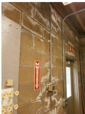
Figure 5. Water damage inside the Headworks Electrical Building
