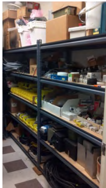
Figure 9. Storage Rack Requires Bracing
