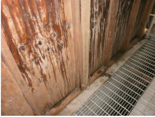
Figure 1. Water damage was observed on the shear walls. The building is not currently anchored down to the slab.
