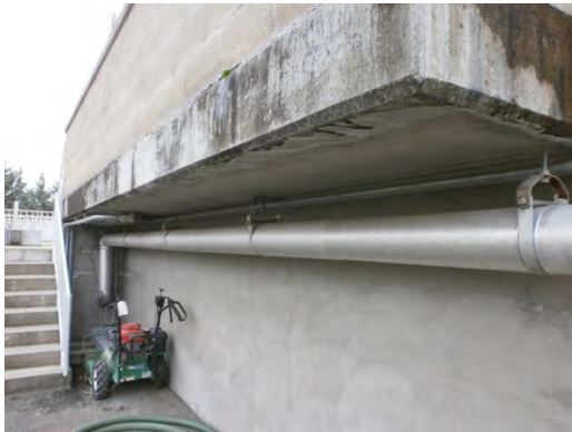
Figure 3. Unbraced piping under the deck. Headworks Structure
