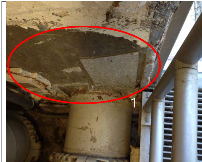
1. Cladding deterioration and exposed wire framework.
