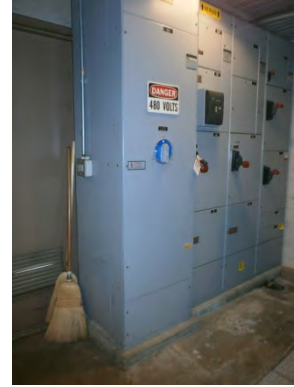
Figure 2. Electrical cabinets are not anchored to the floor.
