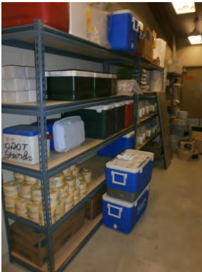
Figure 39. Storage racks are not anchored
