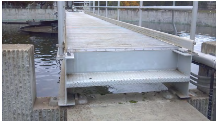
Figure 4. Secondary Clarifier No.3, the bridge walkway bearing requires strengthening.
