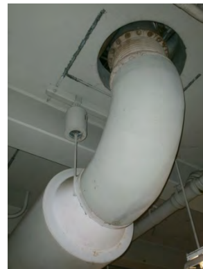
Figure 12 .Silencer without lateral bracing
