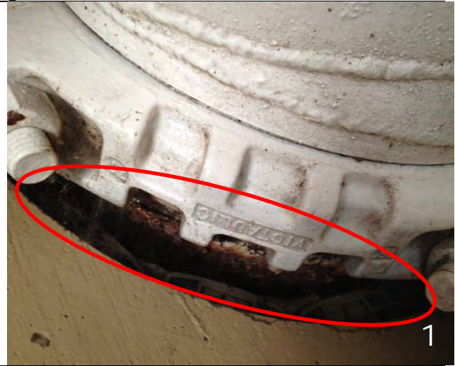
1. Inside wall core rusted.
