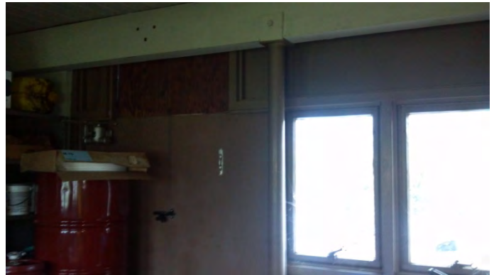
Figure 4. Large opening in the south shear wall of the building.
