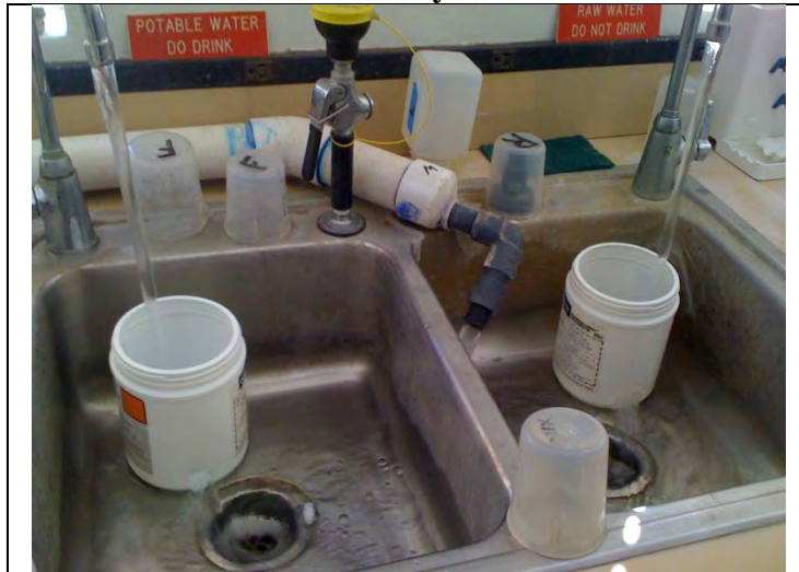
Finished water and raw water taps used for water quality monitoring and analysis.
