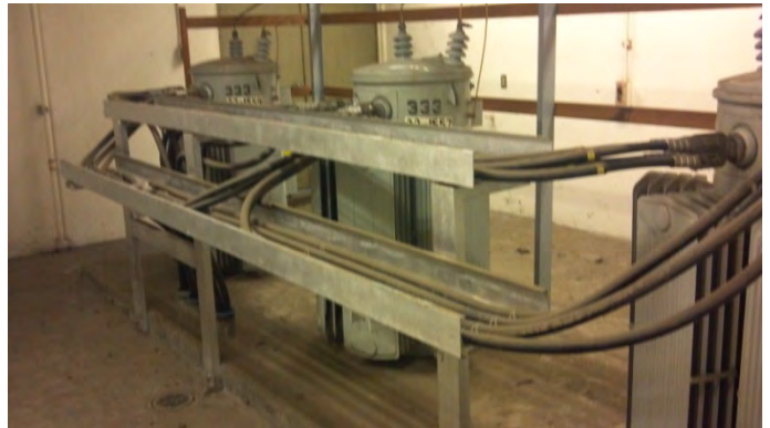
Figure 10.Transformers require to be anchored
