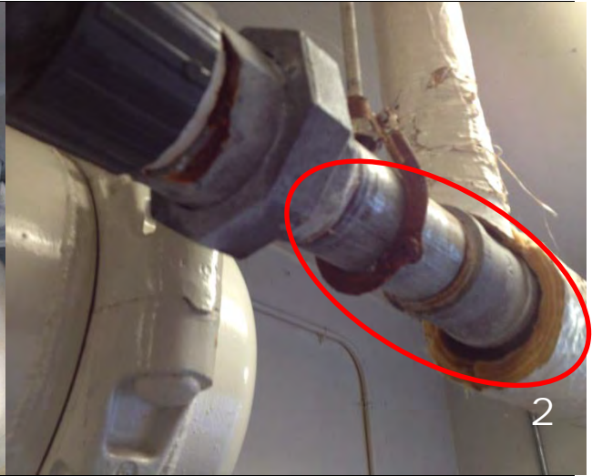
2. Pipe hanger showing signs of rust, pipe not insulated.
