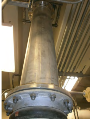
Figure 19. Blower duct is not braced
