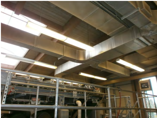
Figure 27. Duct work requires bracing
