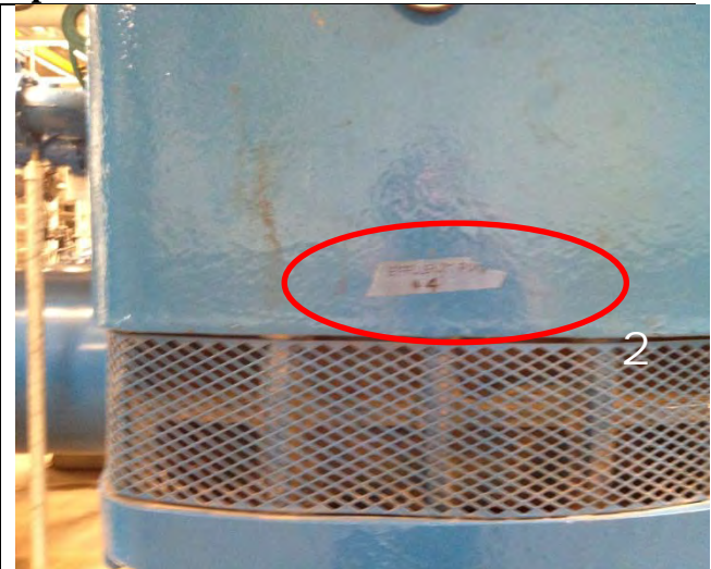
2. Label worn and in need of replacement.
