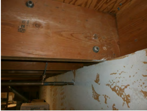
Figure 37. Out of plane anchorage is not provided for the penthouse roof deck.
