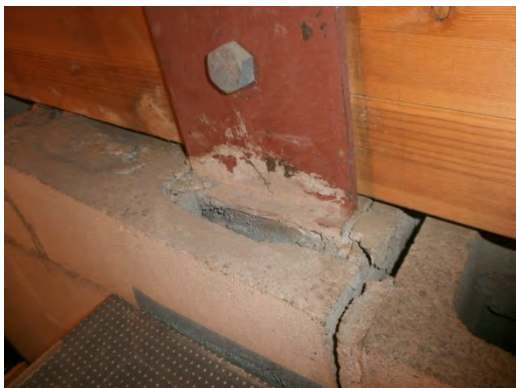
Figure 35. Penthouse crawlspace: The masonry blocks are not fully grouted
