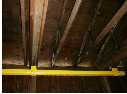
Figure 2. Monorail attached to the roof trusses.
