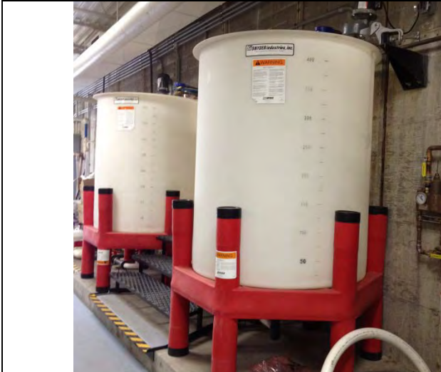
No spill containment for batching tanks.
