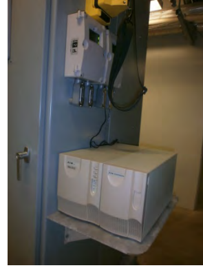
Figure 20. UPS batteries are not protected against lateral loads
