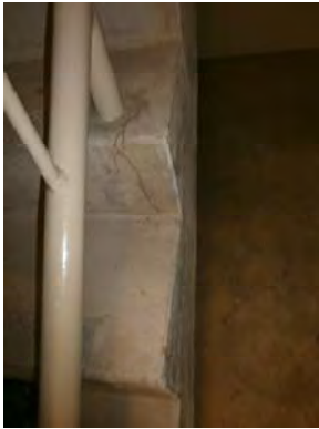
Figure 3. Cracking was observed occasionally on the concrete staircase, at the guardrail post attachment.
