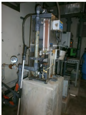
Figure 23. Sampling equipment needs to be braced to the concrete pedestal
