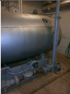
Figure 15. Boiler is not anchored to the floor
