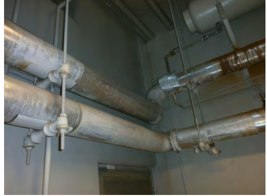
Figure 14 Hot Water pipes are not braced laterally.
