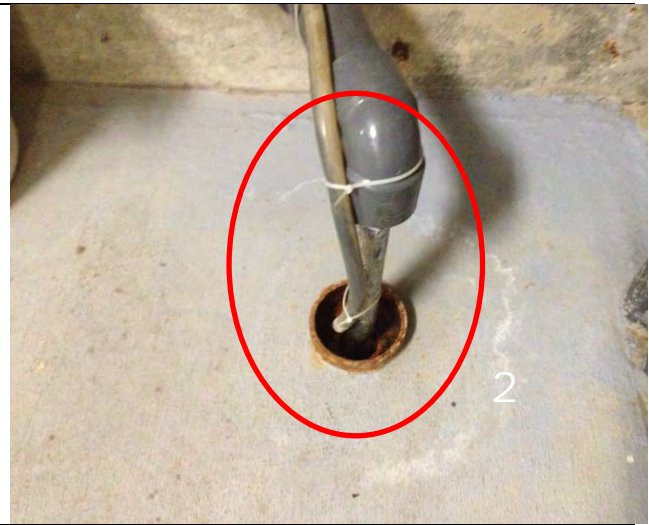
2. Drain may not be adequately sized to handle flows. Drain lines are not seismically supported.
