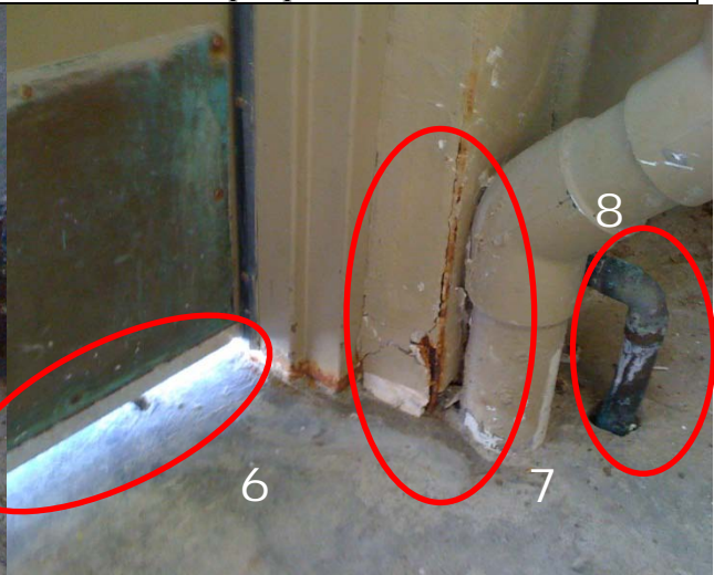
6. Door not sealed: HVAC problem. 7. Door frame rusting and deterioration. 8. Pipe coating corrosion.
