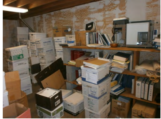
Figure 32. Storage rack in the penthouse is not braced
