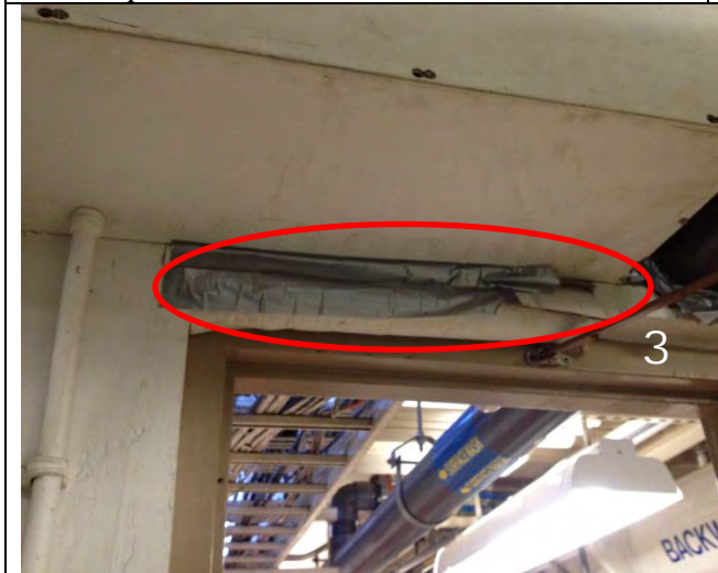
3. Tape and insulation may need to be replaced above doorframe.
