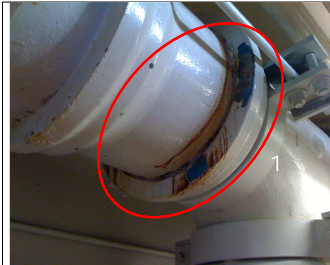
1. Joint experiences intermittent leaking and is corroding.
