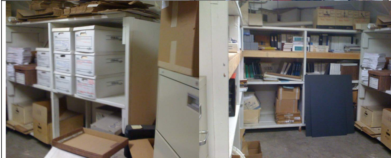
Portions of the HVAC control attic used for storage.
