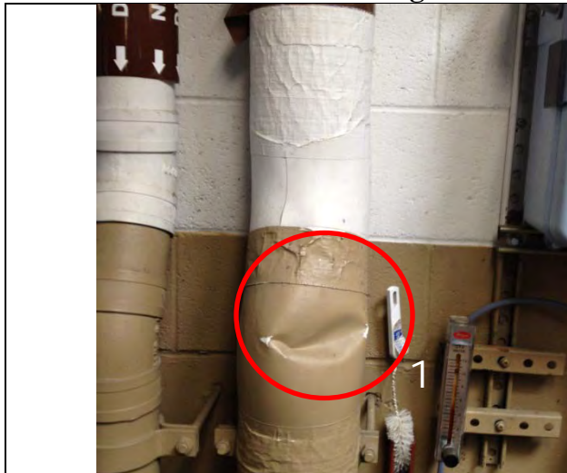
1. Damage to pipe insulation.
