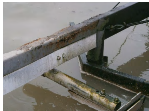
Figure 6. The Thickener mechanism shows signs of wear and corrosion.
