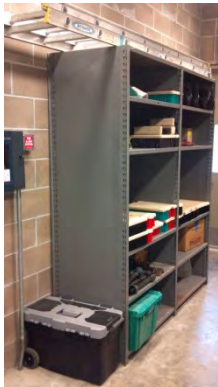
Figure 3. Storage rack in the RAS/WAS electrical room is not anchored
