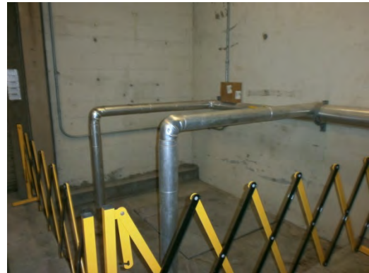
Figure 28. Hot Water piping requires bracing
