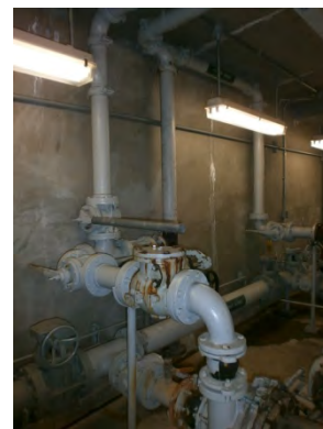
Figure 6. Piping in the basement of the Headworks Electrical Building requires additional bracing.
