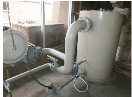
Figure 6. Surge Tank in the Digester Control Building appears to be unanchored
