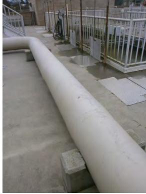
Figure 1. Long run of pipe is not tied to the deck
