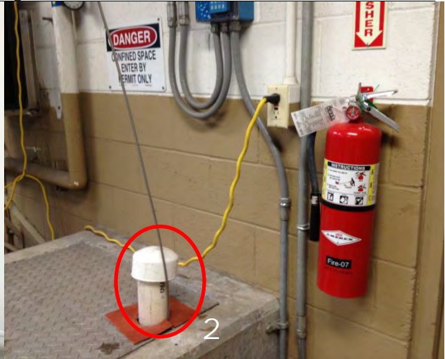
2. Poor access to wet well level
