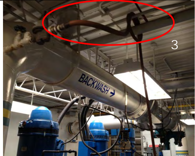
3. Temporary hose connection
