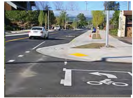
An example of a retrofitted curb ramp to an existing sidewalk
