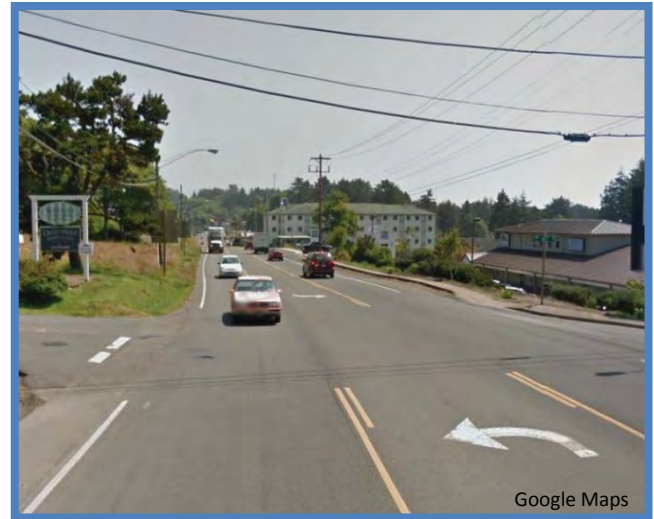
Discontinuous pedestrian facilities along US 101 at NE 36nd Drive
