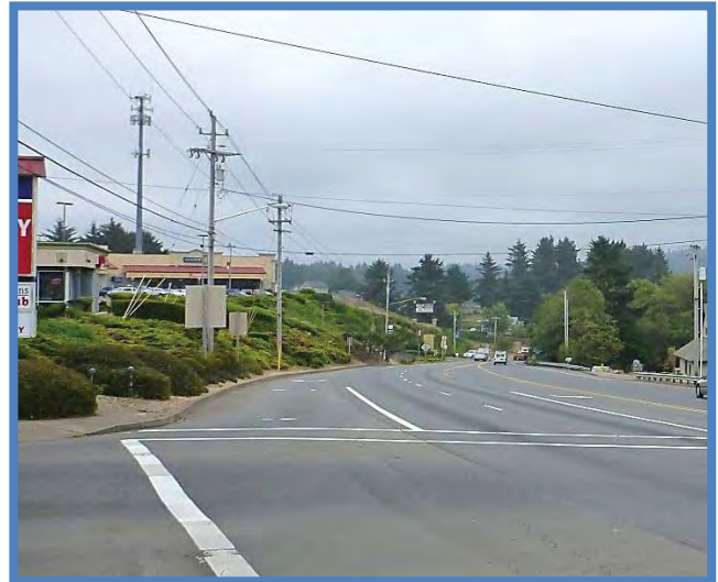
Lack of bicycle facilities at US 101 and Logan Road
