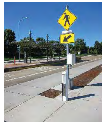
An example of an enhanced pedestrian crossing with a Rectangular Rapid Flashing Beacon
