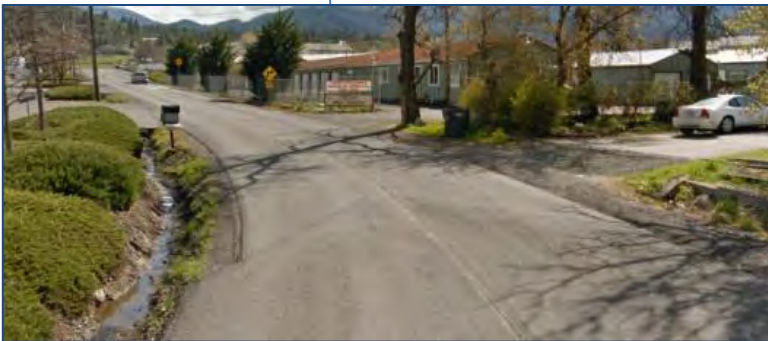
No Curb, Gutter, or Sidewalk
