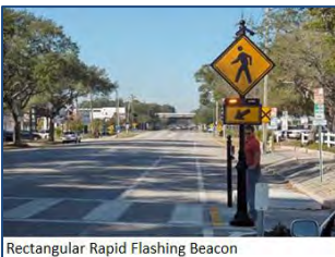
Rectangular Rapid Flashing Beacon
