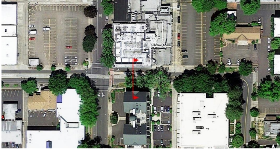
Figure 12: Aerial View of High Street Station. Source: Google Earth Pro
