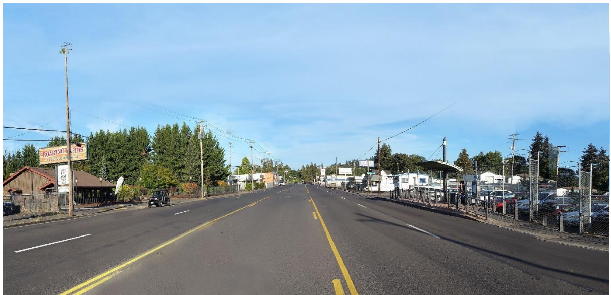
Figure 95: Before Improvements at Lexington Station
