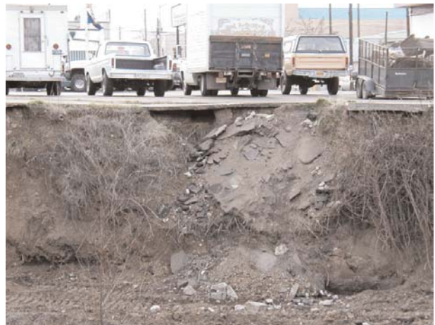
Erosion behind businesses - Central Zone
