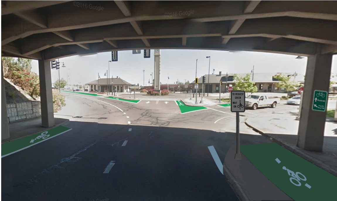
Figure 27: View of new infrastructure for bicycles at underpass leading to the Amtrak station.
