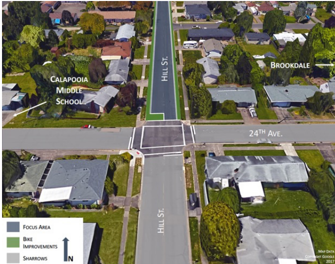
Figure 40: View of Hill Street at 24th Avenue with bicycle infrastructure.
