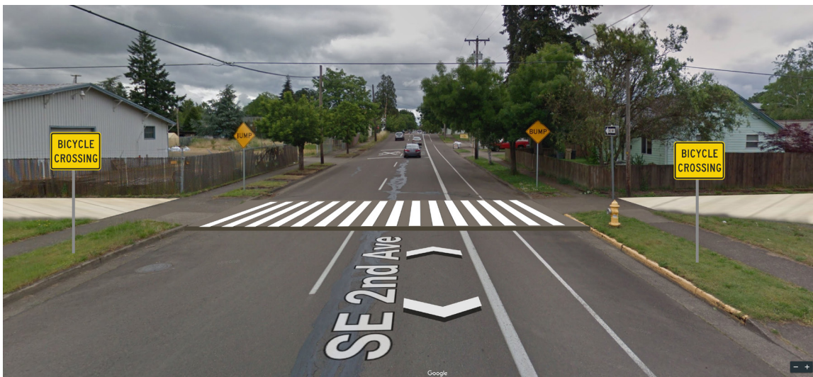
Figure 20: Thurston canal crossing 2nd Avenue after crosswalk addition and signage.
