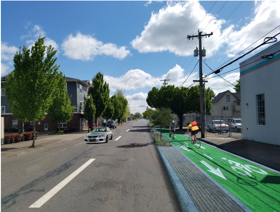
Figure 3: Phase 2 of the street redesign with bicycle infrastructure on First Avenue in downtown Albany includes new bioswales and lane protection.
