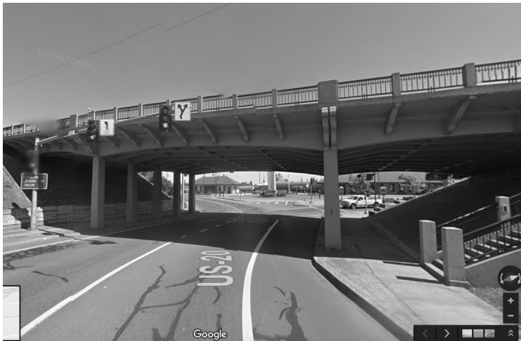
Figure 28: Current view of Lyon Street.
