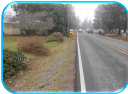
Shoulder and ditch on Leland Road (Segment 3)
