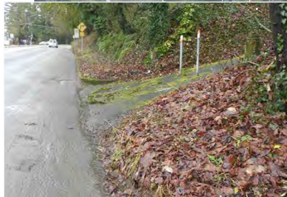
Path connection at 5th Street has no wayfinding signage. In addition, lack of landing and steep slopes are a hazard for path users.
