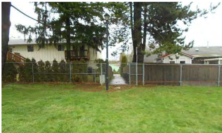
Sidewalk ends at fence with 2-ft wide gap (limited accessibility)
