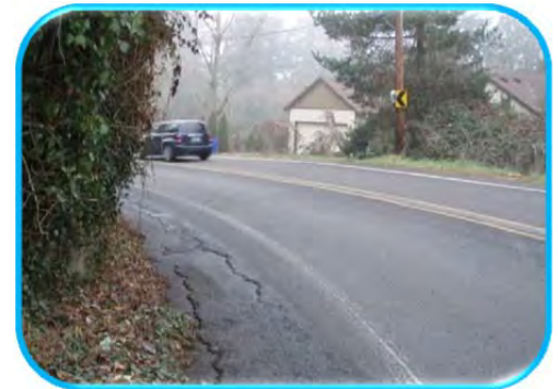
Tight turn on Linn Avenue between 4 th Street & Oak Street
