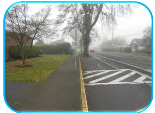
Midblock crossing at former Mt. Pleasant School
