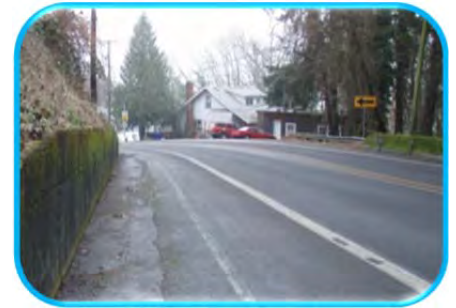
Retaining wall and jersey barrier on Linn Avenue (Segment 1)
