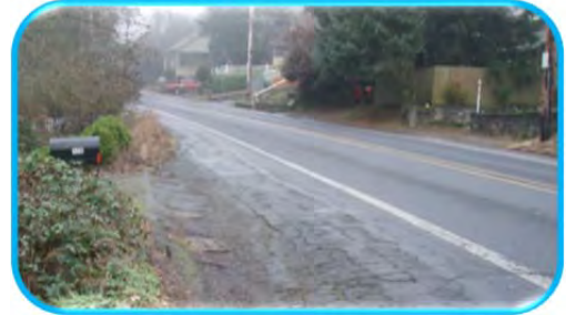
Pavement conditions in shoulder of Linn Avenue
