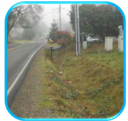
West shoulder on Leland Road
