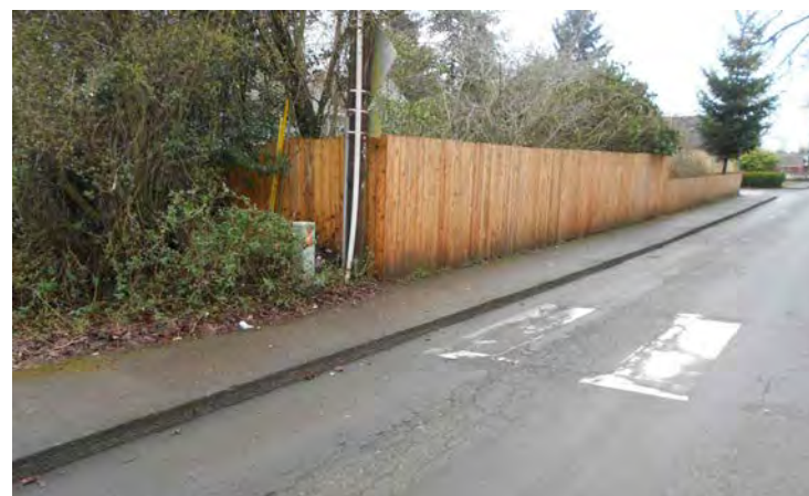
Crosswalk from neighborhood lacks sidewalk landing
