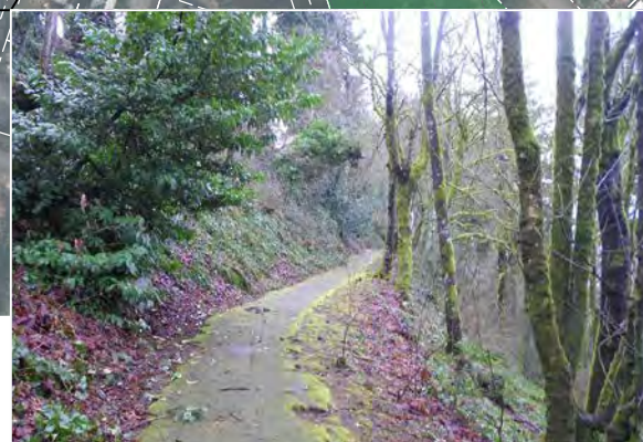
Existing asphalt path is deteriorating in some locations and is not ADA compliant
