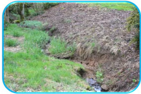
Soil erosion in Singer Creek Park
