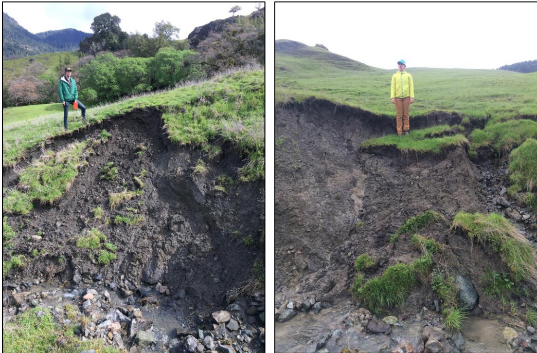
Photos 1 and 2: bank failures in a channel coupled with the Twin Towers slide (figure 10). Photos taken in late March, 2017, after heavy rain.
