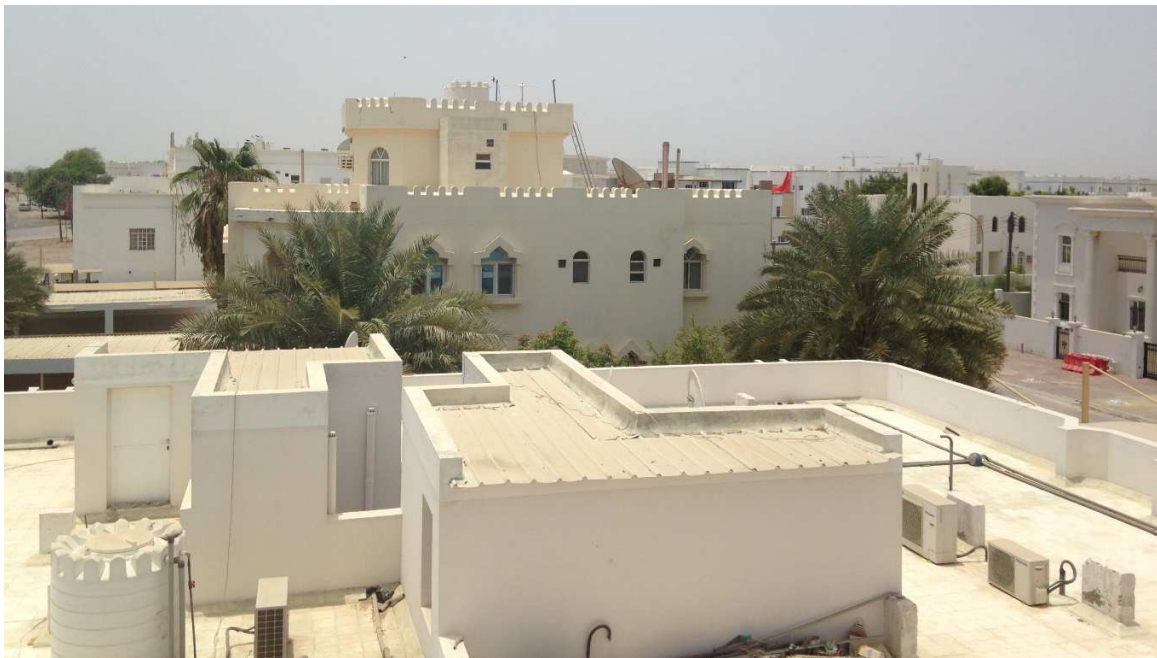
Photo 5.4: Homogenised architecture to resemble forts; Al Hail, Seeb.
