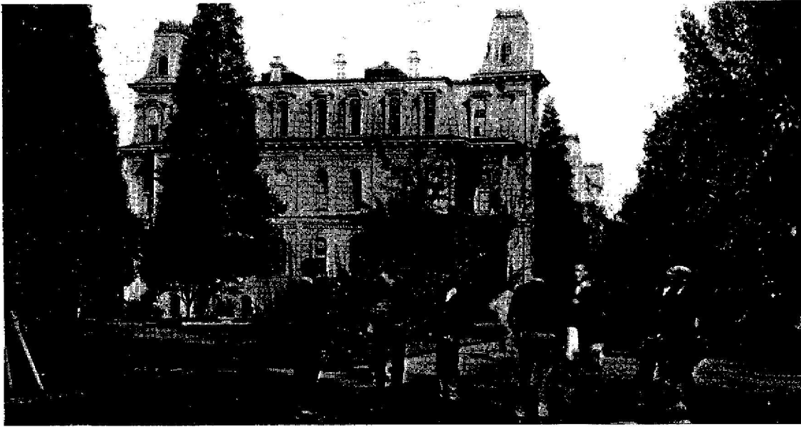
Before "Old Deady's hallowed hall"
