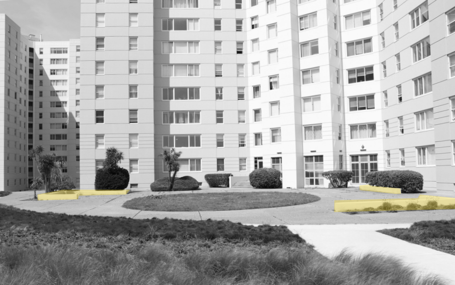
Figure 4.14 Existing staggered concrete forms (March 20180.
