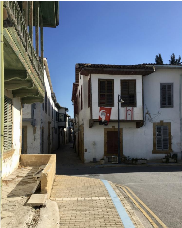
Figure 5.9 Ottoman cumba and broad eaves seen on single-family homes in the Arabahmet neighborhood. Photograph by author, December 2017.
