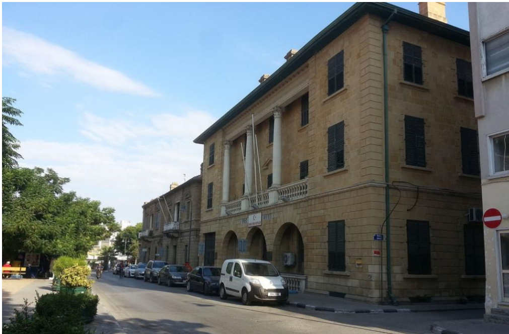
Figure 3.8 Nicosia Post Office, built 1925. Source: Seksen iki yüz kırk beş, The historical, neo-Renaissance style post office in Sarayönü, North Nicosia, Northern Cyprus , 2015, Wikimedia Commons.
