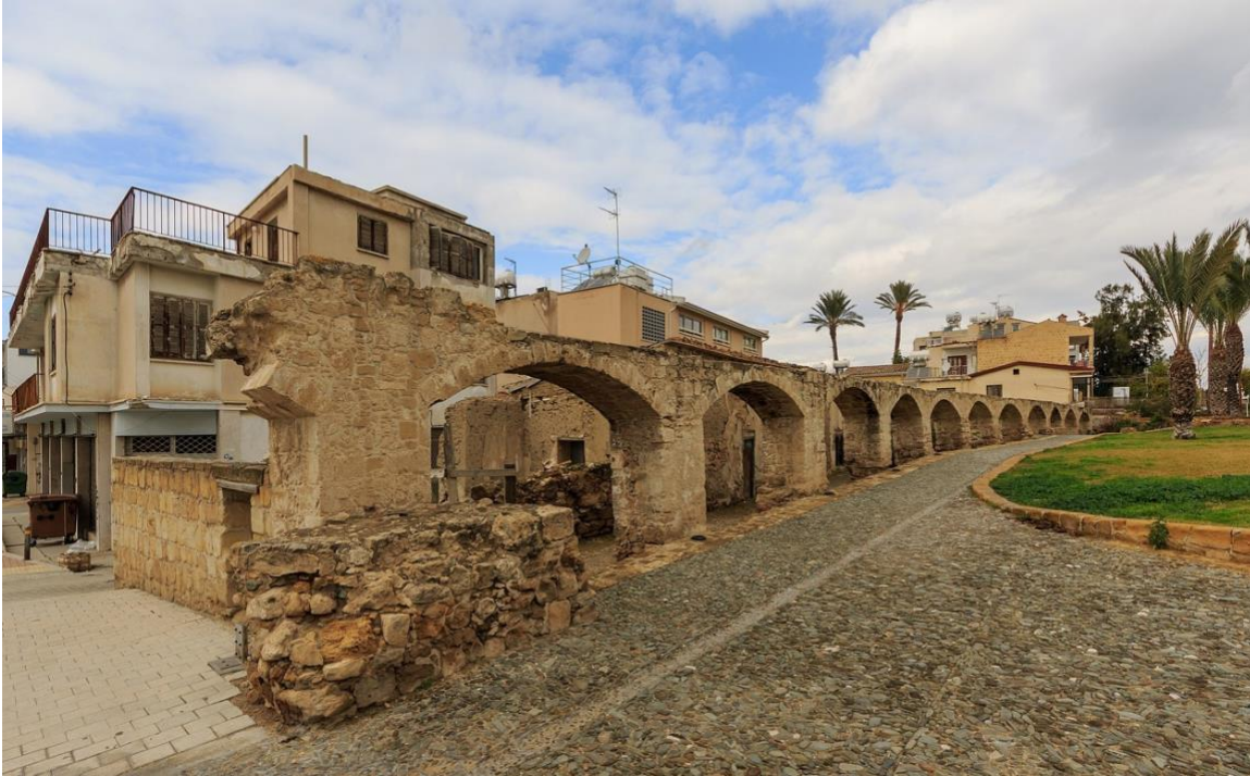
Figure 3.1 Roman Aqueduct in East Nicosia. Source: Alexander Savin, Old Aqueduct in Nicosia, Cyprus , 2017, Wikimedia Commons.
