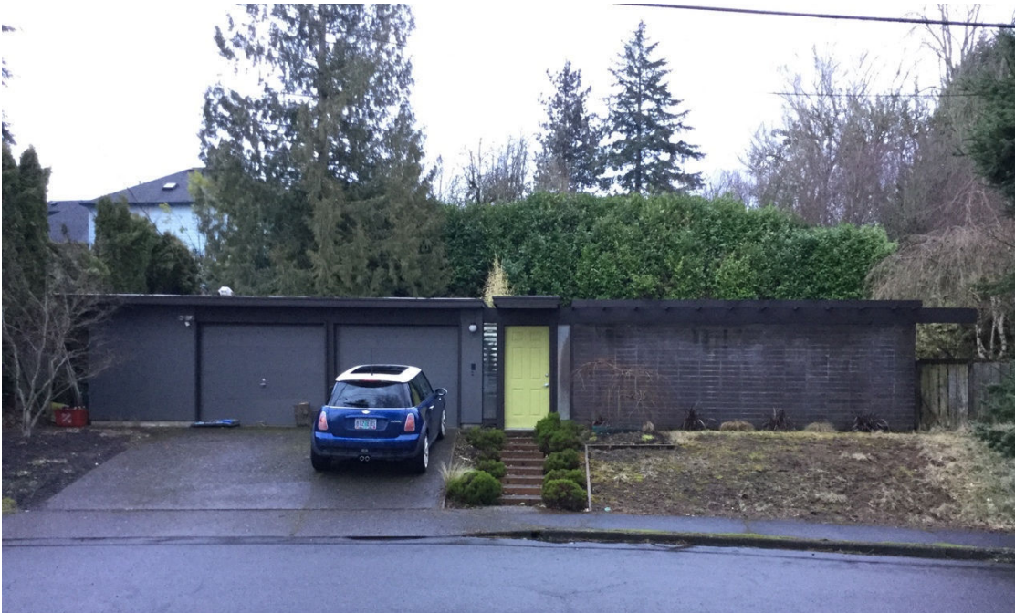
Figure 66: 8580 Southwest Cecilia Terrace, facing northwest (Samantha Gordon, February 28, 2017).
