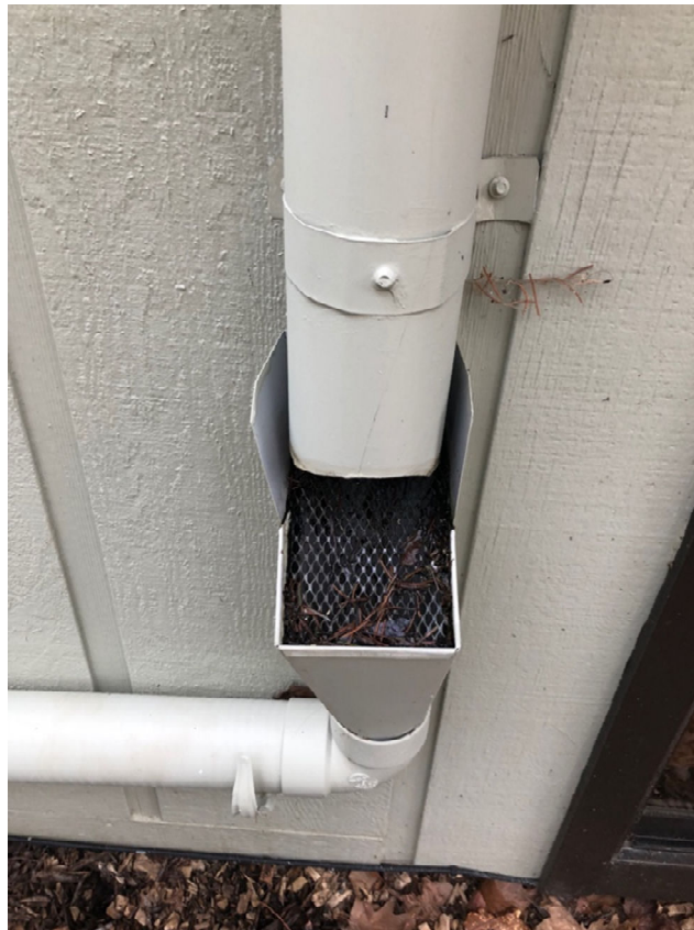
Figure 35 - Downspout and drainage join detail, south façade.
