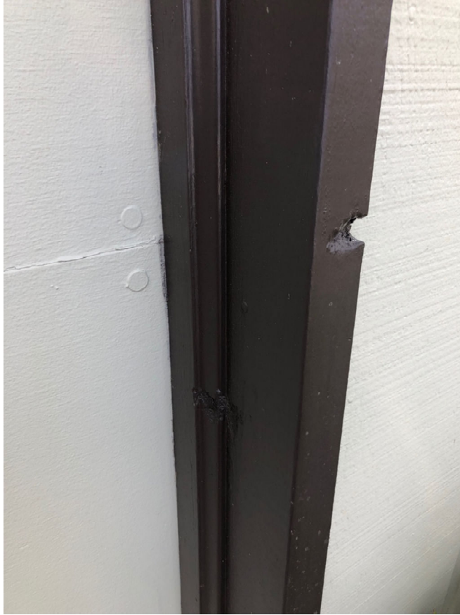
Figure 38 - South garage door and frame detail, west facade.
