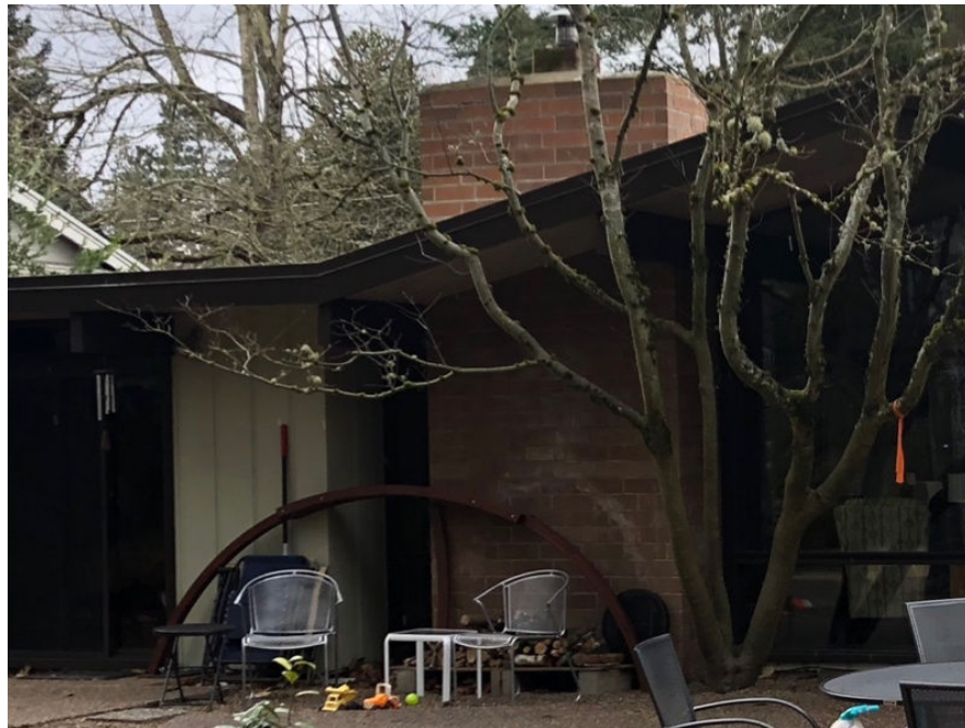
Figure 33 - Chimney, east façade facing west.
