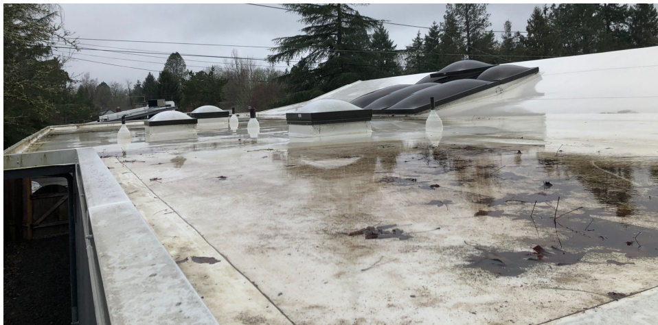
Figure 18 - Skylights on roof, south façade facing west.
