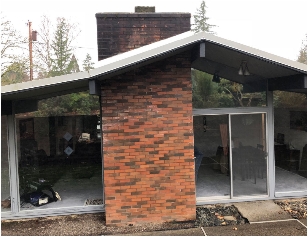
Figure 17 - Chimney, east façade facing west.
