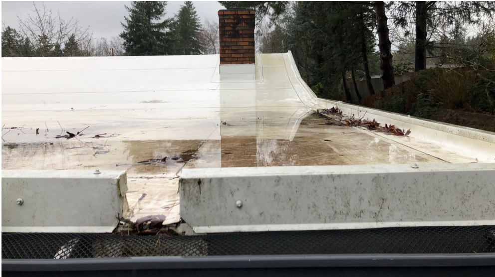
Figure 15 - Metal roofing, east parapet, and south chimney flashing, south and east façades facing north.
