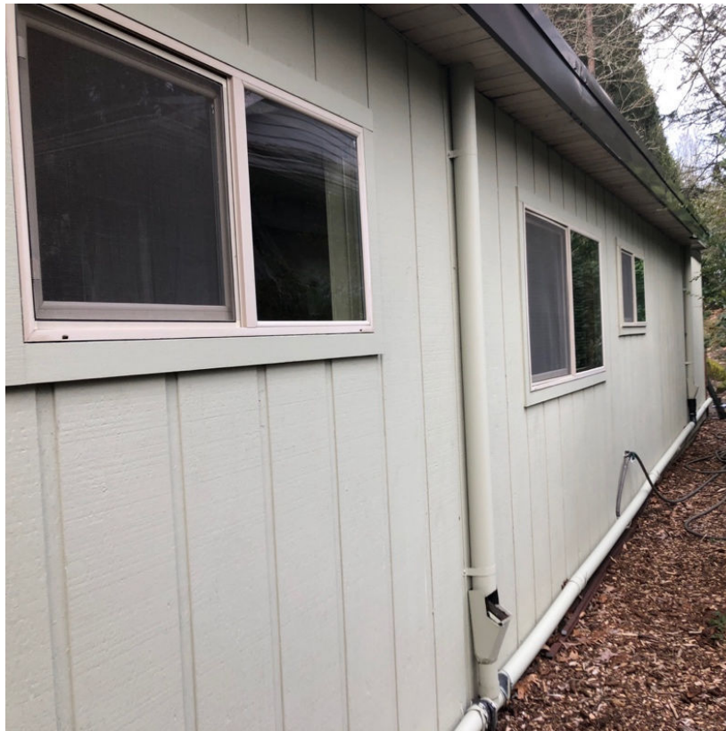
Figure 36 - Siding and windows, south façade facing east.
