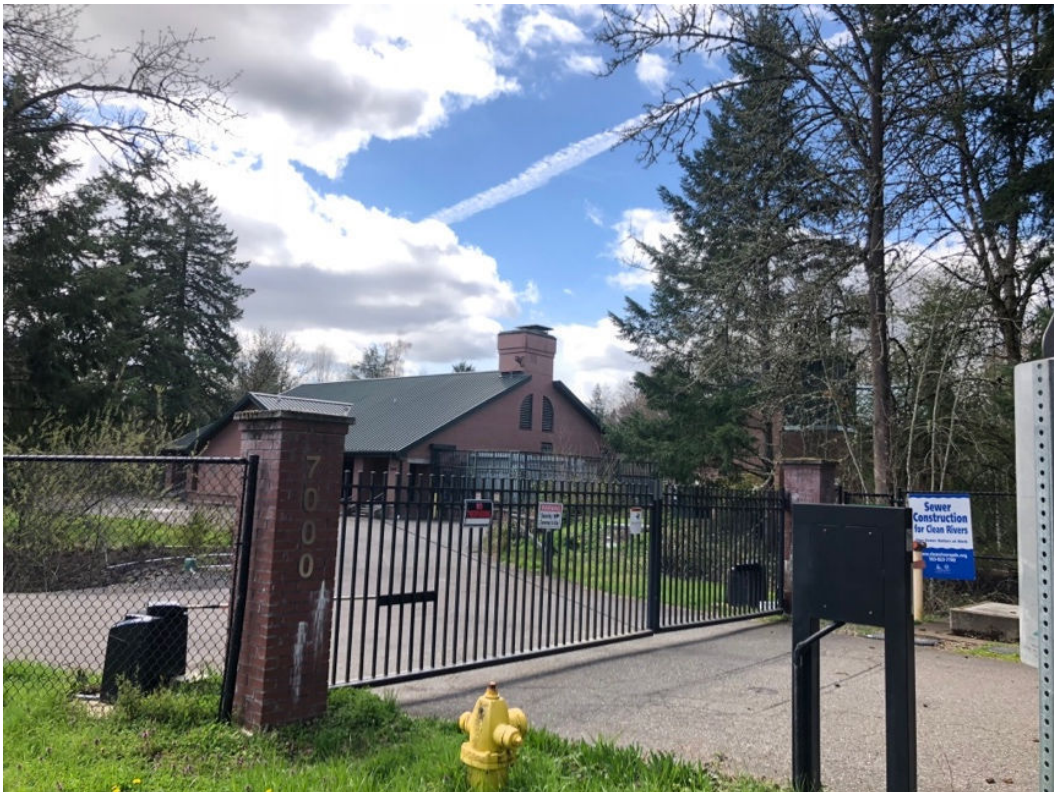
Figure 52 – Entrance to original Fanno Creek Pump Station construction, facing south.
