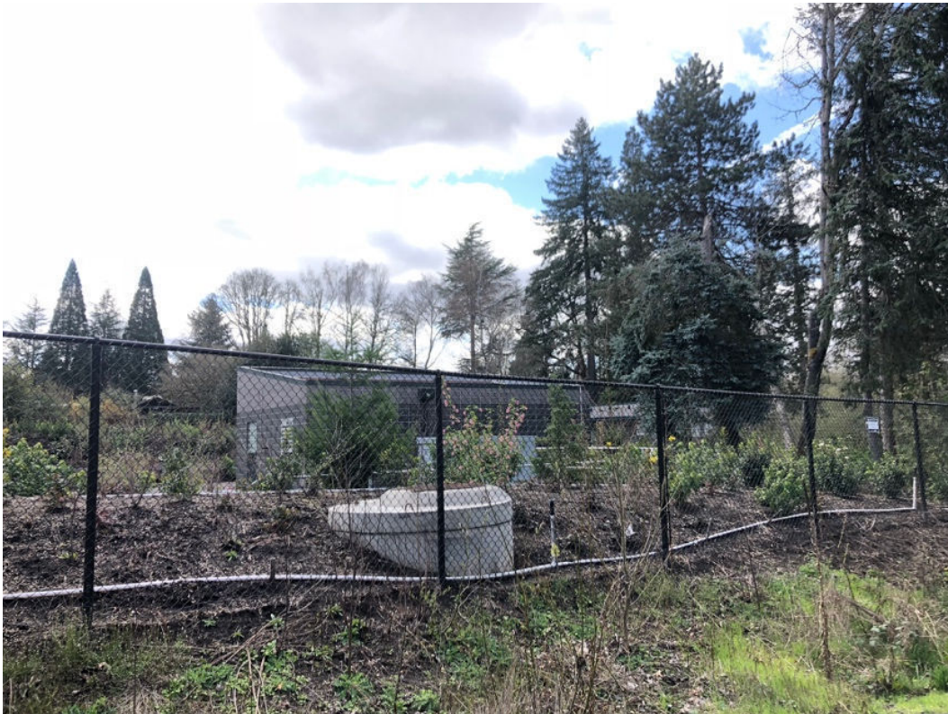
Figure 48 - View of second set of Fanno Creek Pump Station buildings from Fanno Creek Trail, facing southwest.
