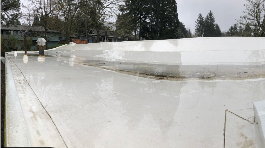
Figure 14 - Metal roofing and vents, north façade facing east.
