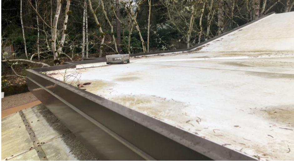
Figure 31 - Membrane roofing and vents, north façade, facing southeast.
